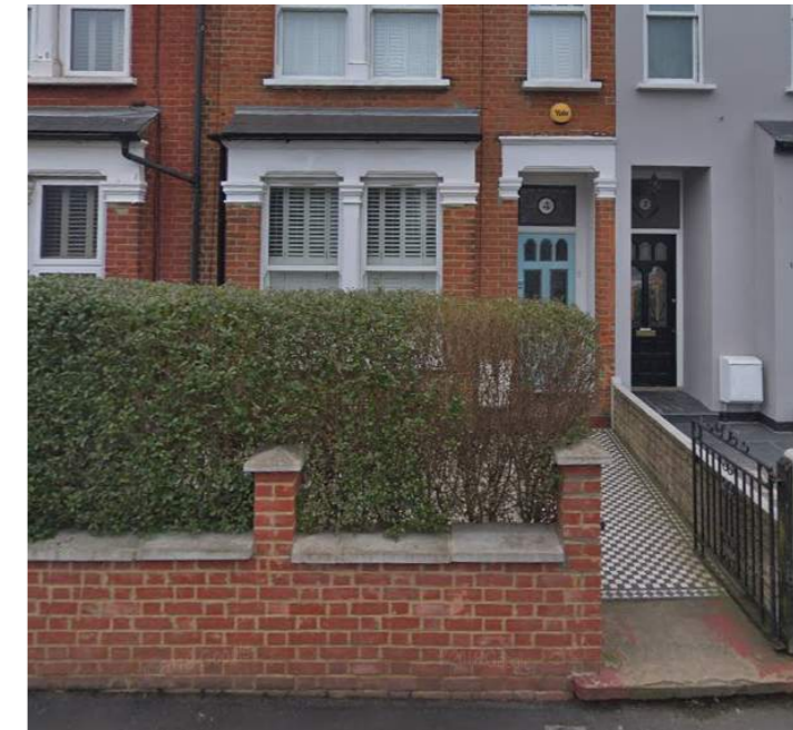
Front Boundary Wall at Lion Road, Twickenham
