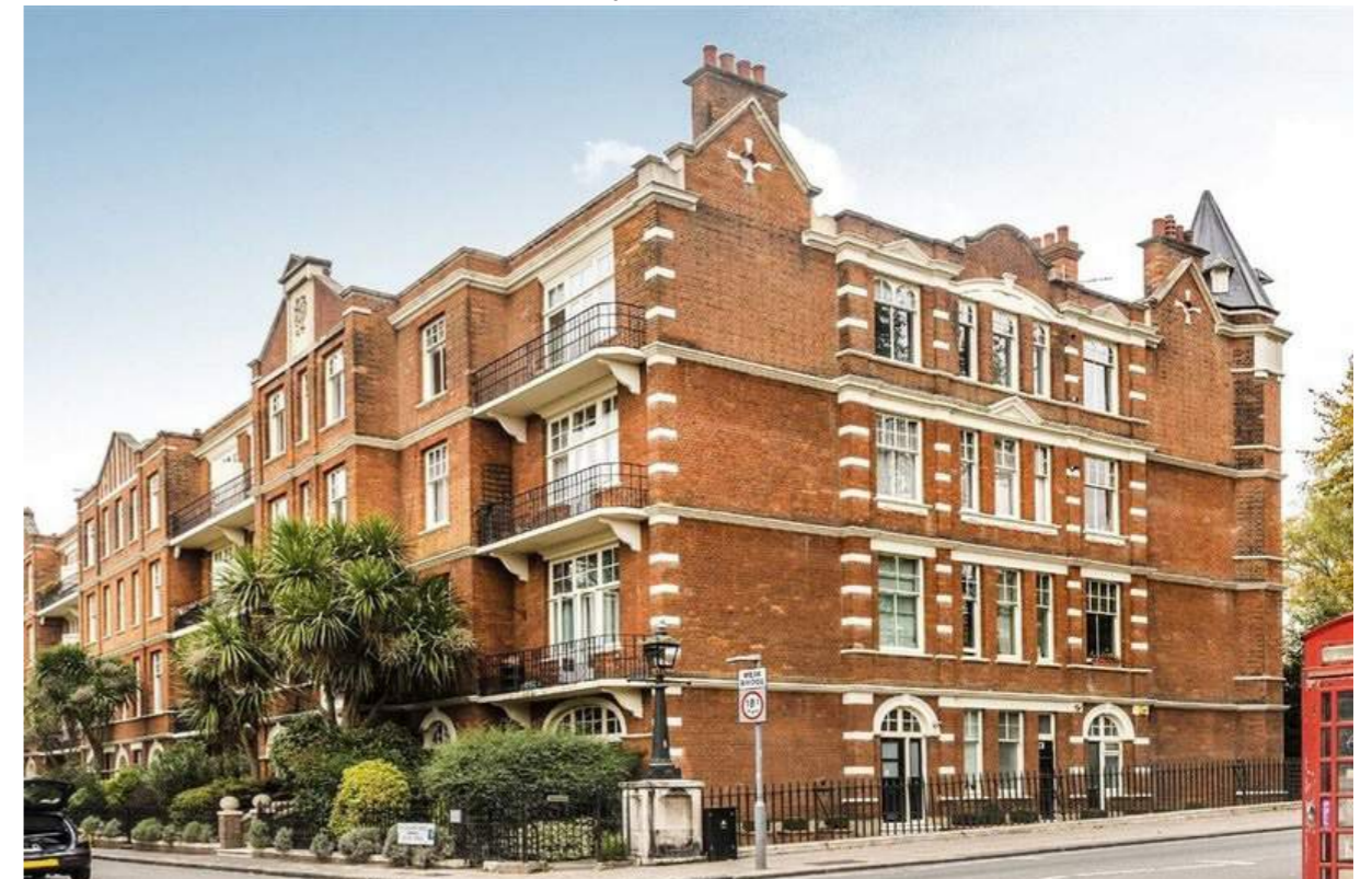
Mansion Block in Willoughby Road, Twickenham
