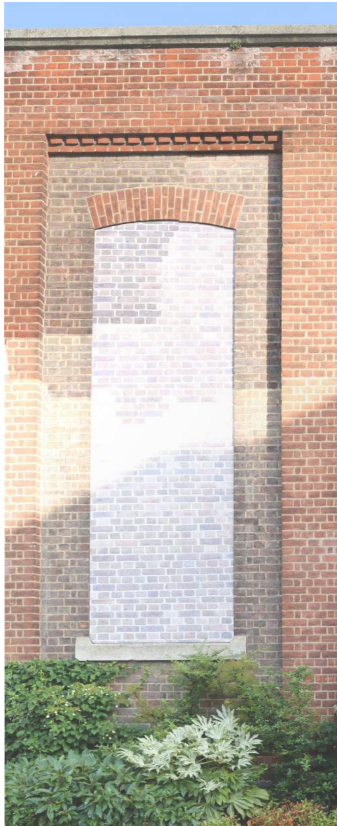
Brick Detailing on Brewery Lane
