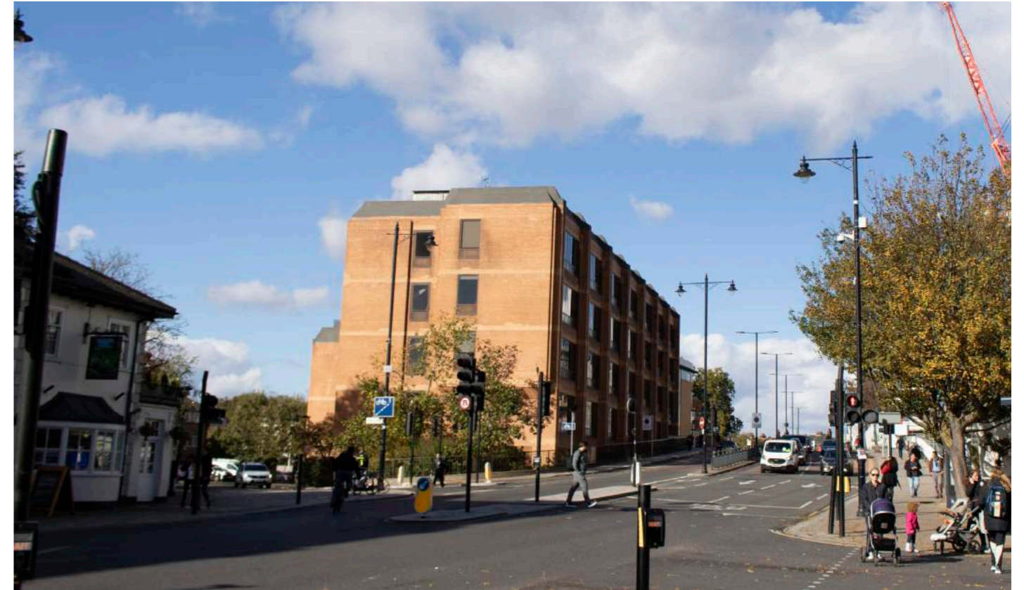
Photo as existing
