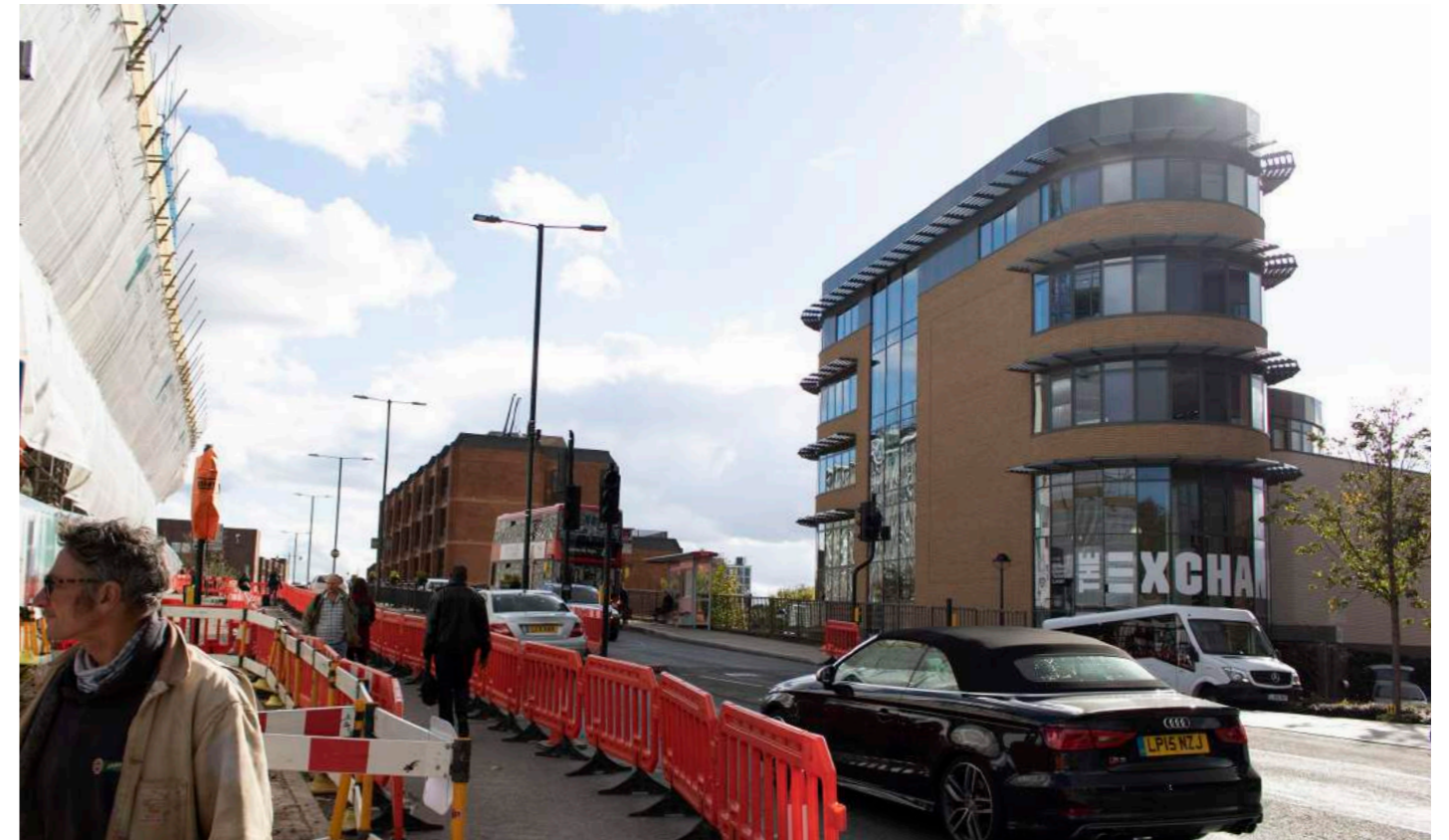
Photo as existing
