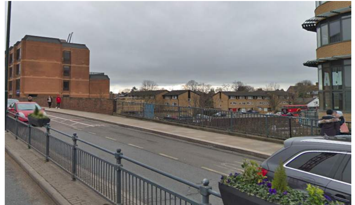
Photo as existing
