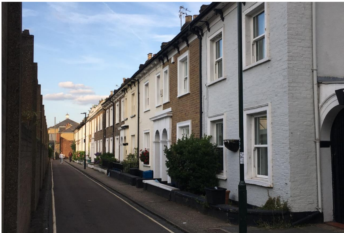
Figure 11: No. 1-16 Mary's Terrace
