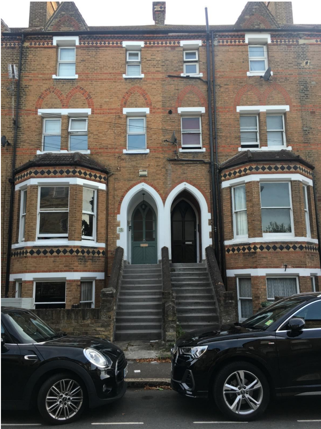
Figure 4: Houses on Queen's Road showing polychromatic detailing
