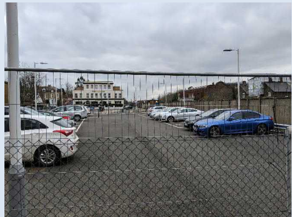
The Site facing southwest. The asphalt surface appears to be in good condition.
