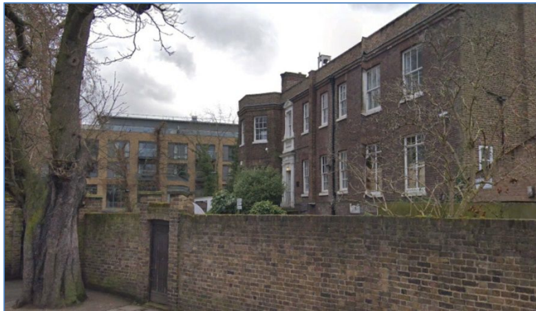
Figure 6 View from Heatham House towards PDA (not visible) (© Google)
