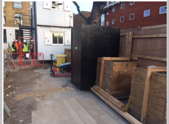
Robust hoarding and temporary concrete ground protection
