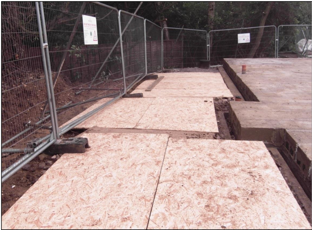
Fig. 1 Ground protection – hoarding over sharp sand and wood chip
