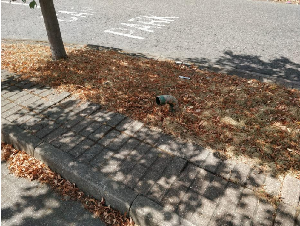
Photo 5: Vent pipe assumed to be associated with possibly identified interceptors
