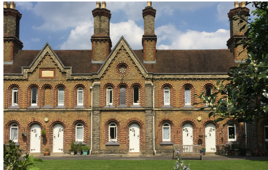
Detailed brickwork surrounds on Almshouses on Sheen Road
