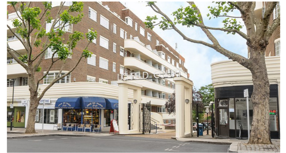
Lichfield Court, Richmond
