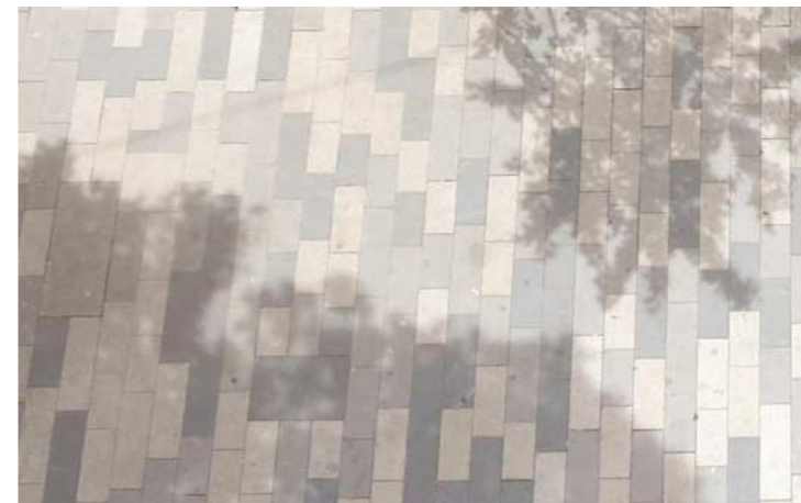
Granite setts (Coloured mix)
