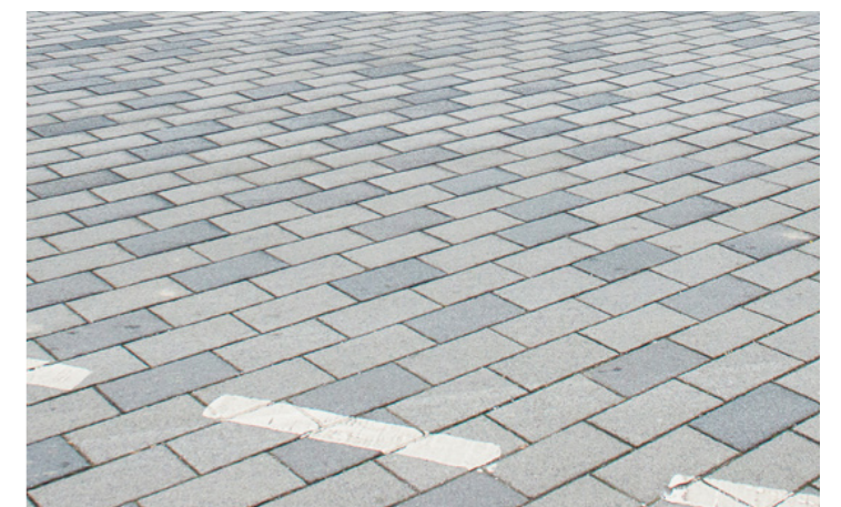
High quality block paving
