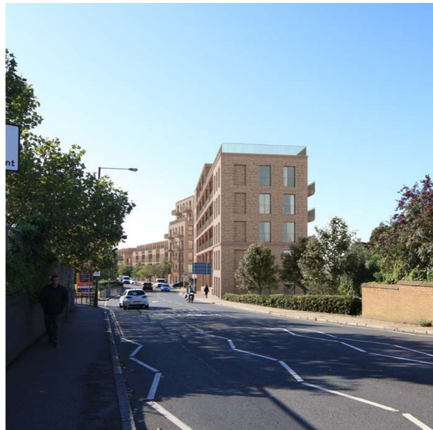
View of building E from Manor Road (looking south)
