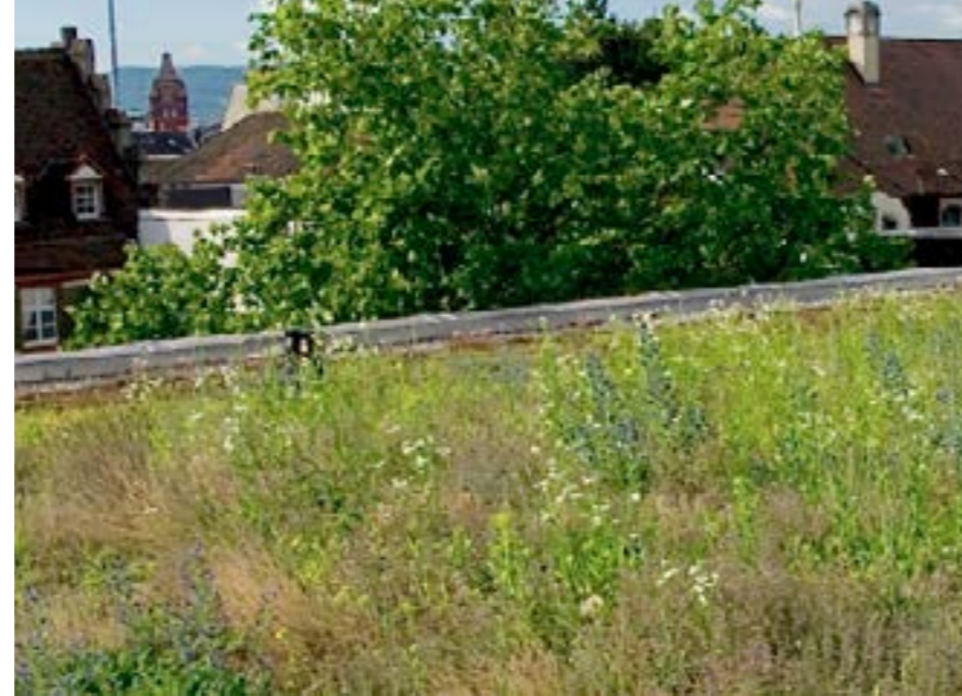
Example of extensive green roof.
