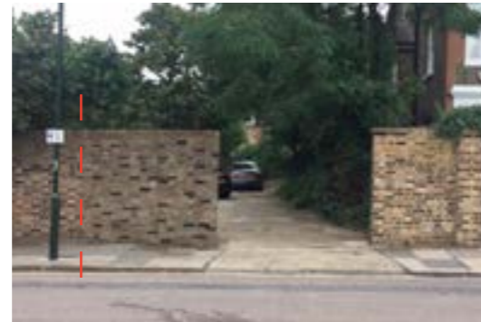
Site access with modern section of brick wall.
