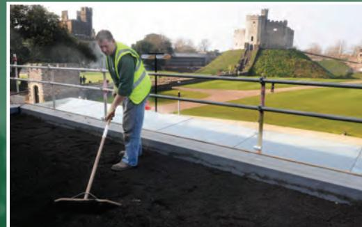
■ Spreading loose substrate
