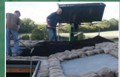
■ Mixed substrate - bagged and loose substrate combination
