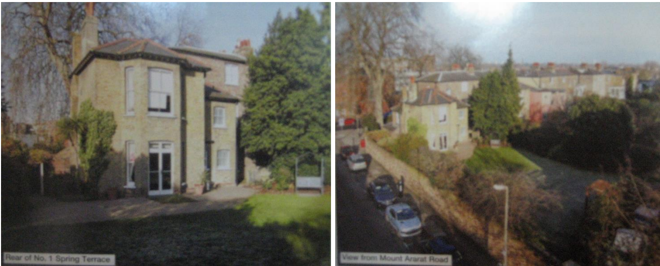
Figure 25: Photographs of the rear of no. 1, featuring on an estate agent’s brochure advertising both no.s 1 and 2 Spring Terrace (“Currently used mainly as Offices”; “Each Building subject to a Commercial Lease expiring May 2015”). Undated, but likely 2010-15.
