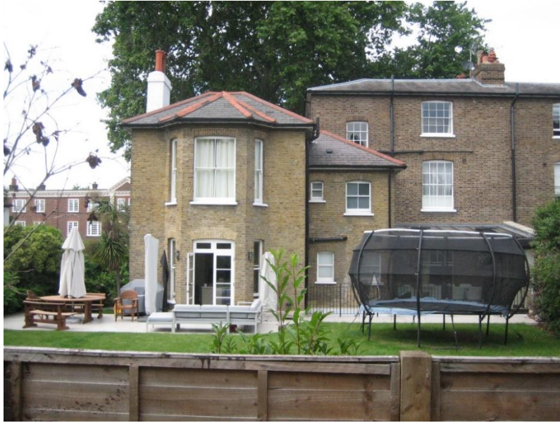
Figure 34: Rear elevation of no. 1 Spring Terrace.
