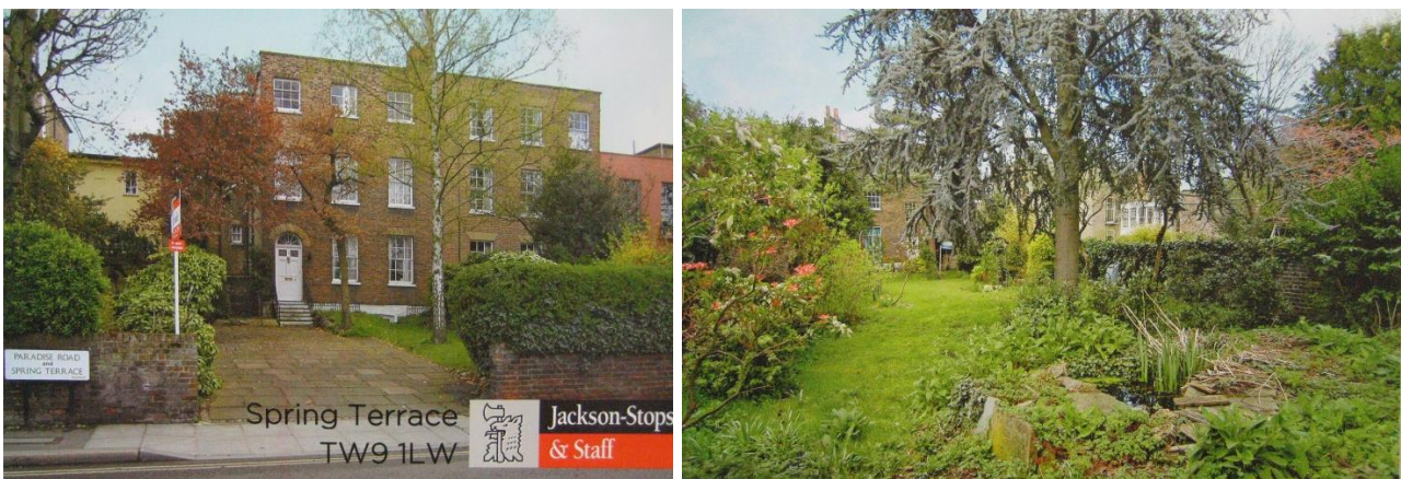
Figure 23: Photographs of the front and rear of rear of no. 2 Spring Terrace featuring in an estate agent's brochure (Jackston-Stops & Staff), 2011.
