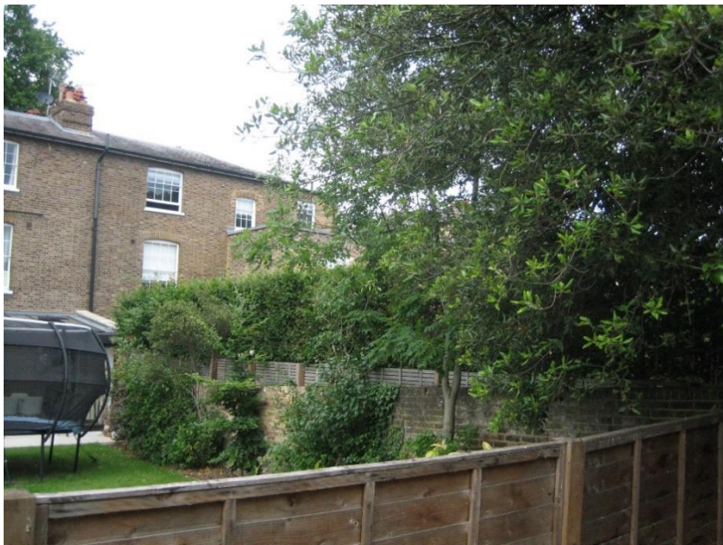
Figure 35: Rear elevation of no. 2 Spring Terrace, viewed from the west side of the subject site.
