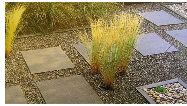
DETAIL OF 450 X 450 MARSHALL UTILITY RICHMOND BUFF PAVING LAID IN PEA GRAVEL
