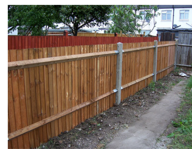
DETAIL OF 1.2m TIMBER ARRIS RAIL FENCE
