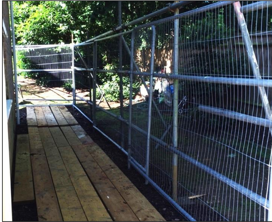
Scaffold board pedestrian ground protection
