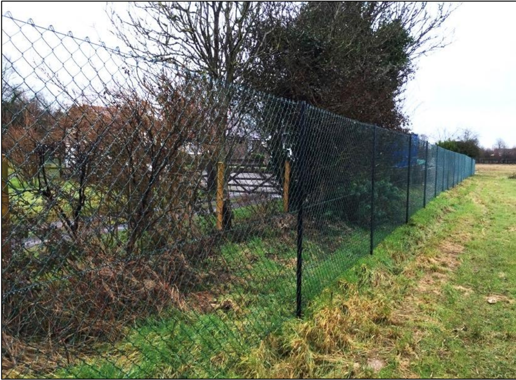
Chain-link on angle-iron uprights
