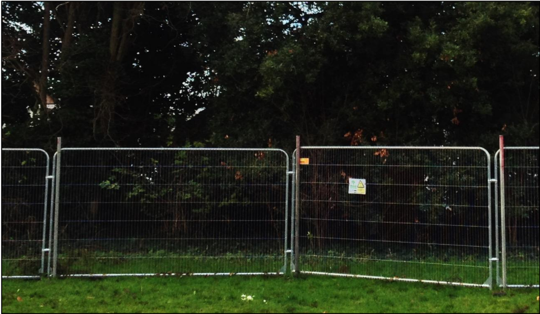
Weld-mesh panels on scaffold uprights
