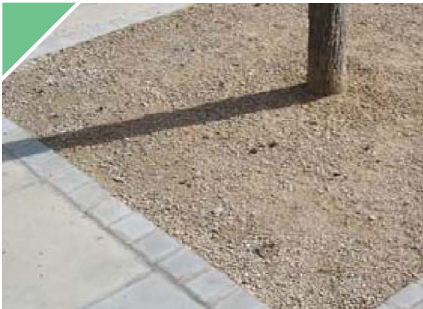
Resin bound gravel tree pit
