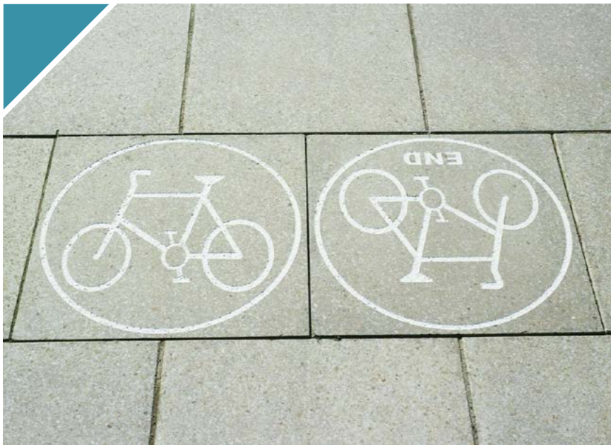
Artificial Stone Flag Paving
