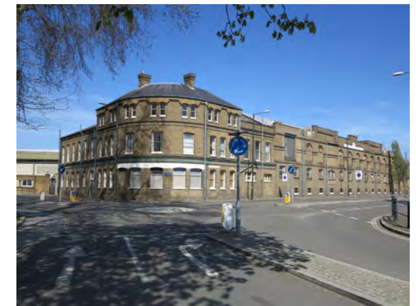
Existing former hotel and Bottleworks Building
