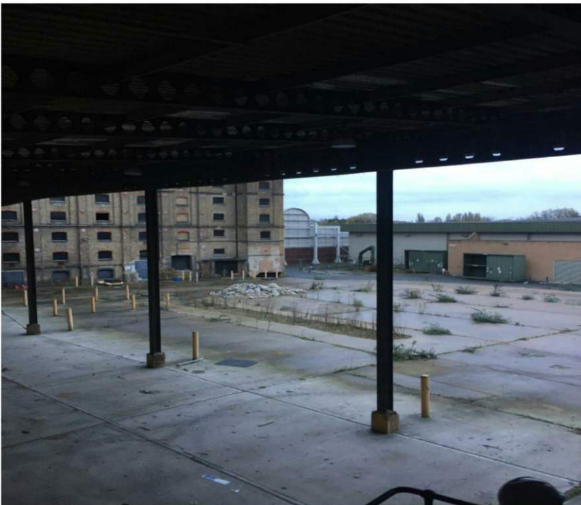
Figure 26 – Additional view towards the back of the Maltings Building
