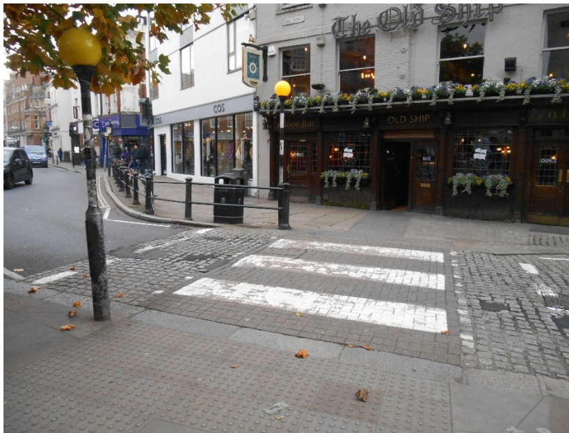
Tactile paving, flush footway surface and raised table.
