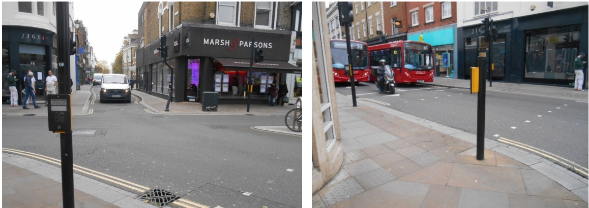
Tactile paving, flush footway surface, sufficient pedestrian waiting space.
