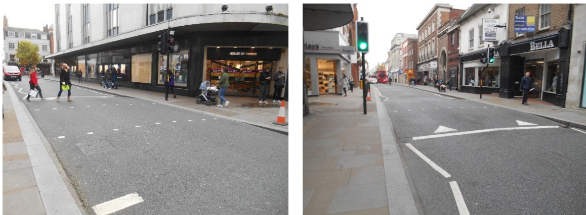
Tactile paving, flush footway surface, raised table, sufficient pedestrian waiting space.
