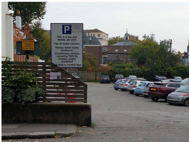
Road sign reads: "CAUTION: Uneven surface in car park".
