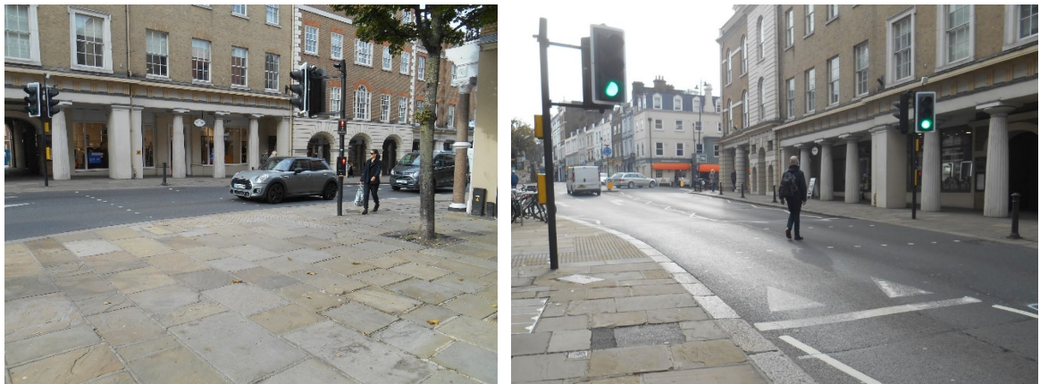
Tactile paving, flush footway surface and a raised table.
