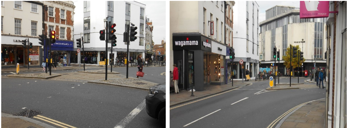
Tactile paving, flush footway surface and raised table.
