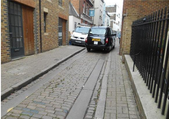
Footways and carriageway are narrow and in a poor condition in some locations
