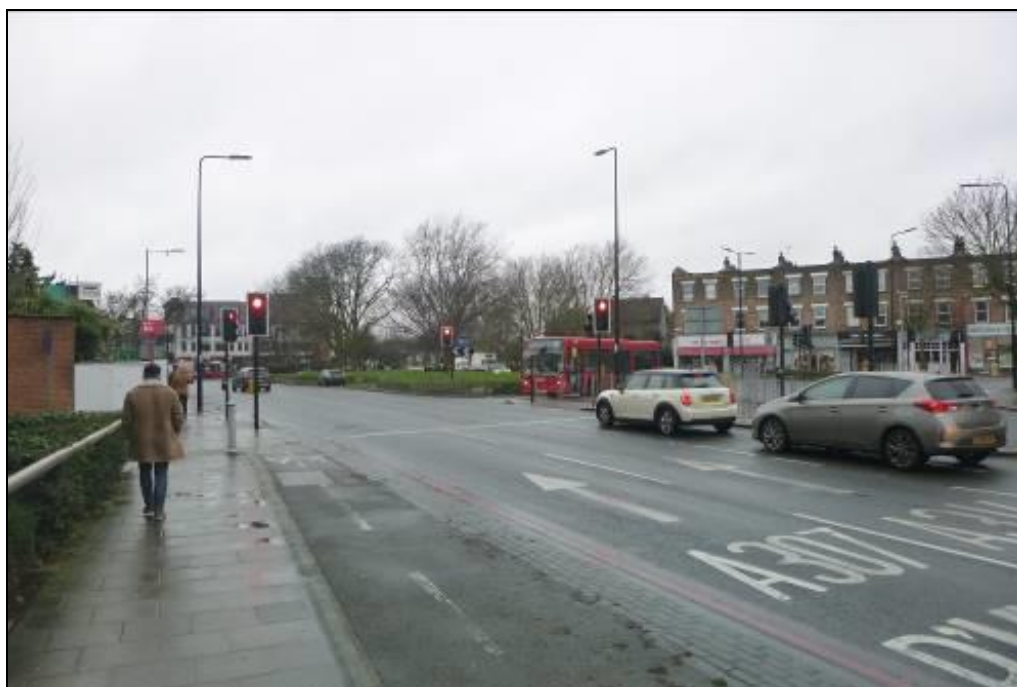
Photograph 6 Showing the roundabout to the southwest
