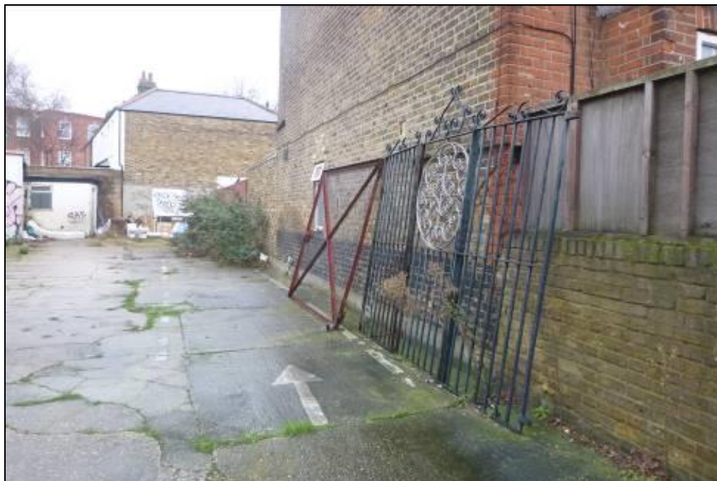
Photograph 3 Showing the site and the adjacent dwelling to the northeast
