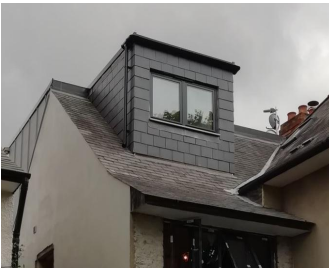
Figure 1: Photo of as-built front dormer
