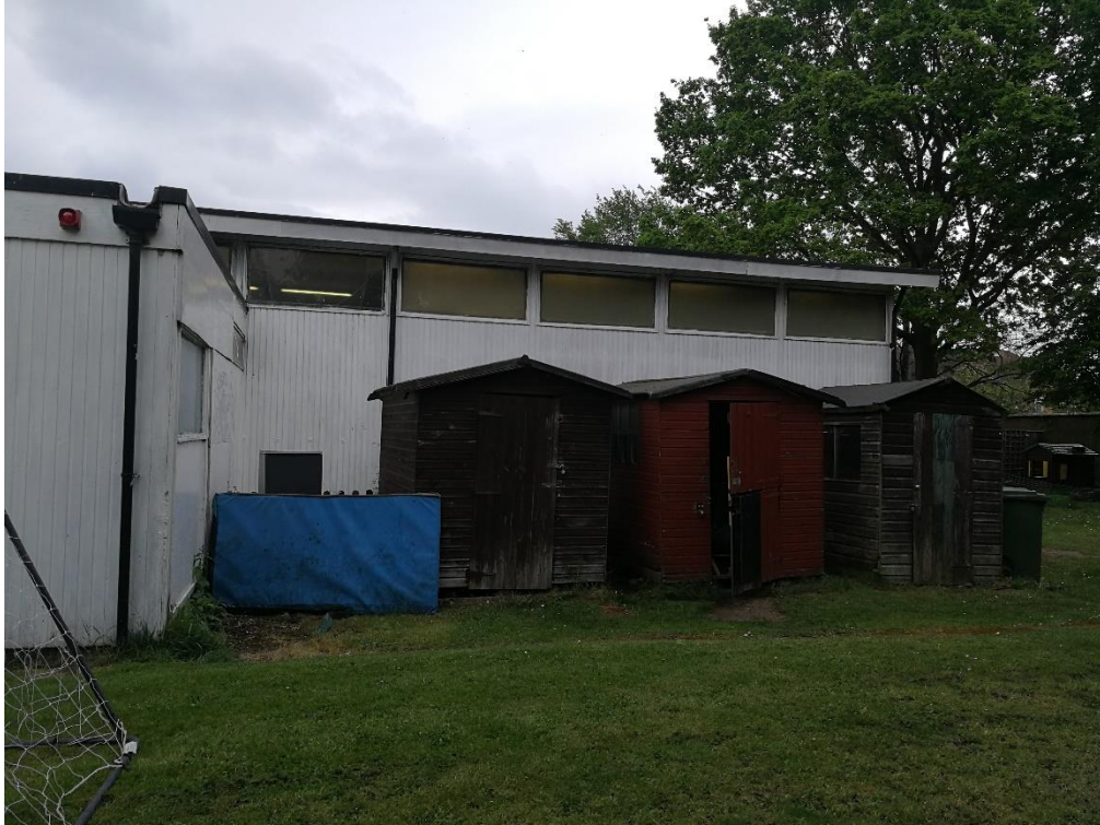
Photograph 6: View of Building 6, the large nursery building in the southern end of the Application Site accompanied by the three small wooden sheds (Buildings 7, 8 and 9).
