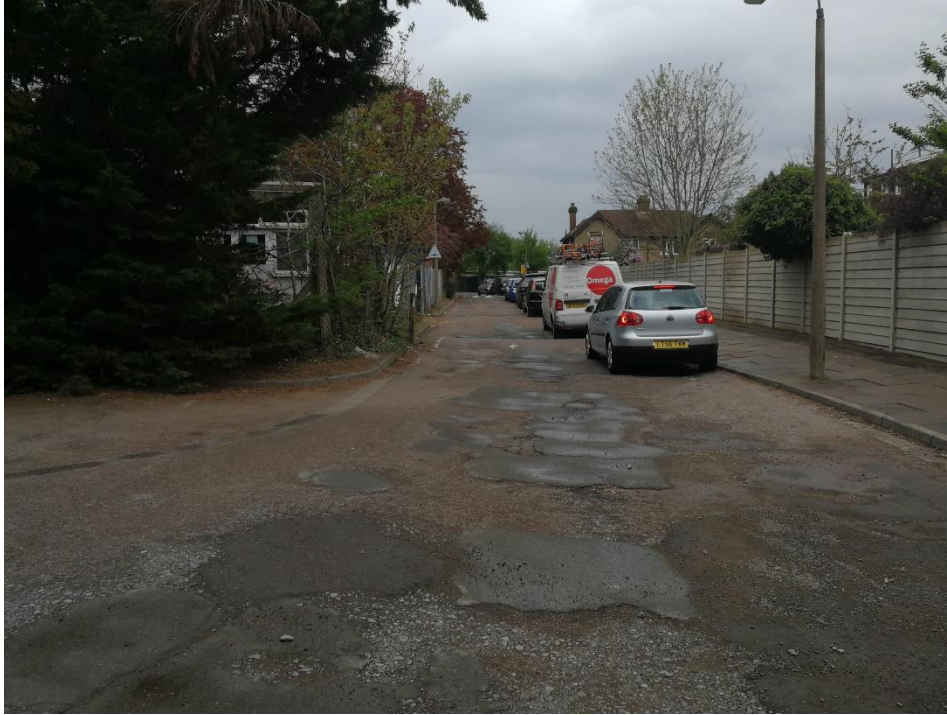
Photograph 8: View of hardstanding at the eastern edge of the Application Site looking north.
