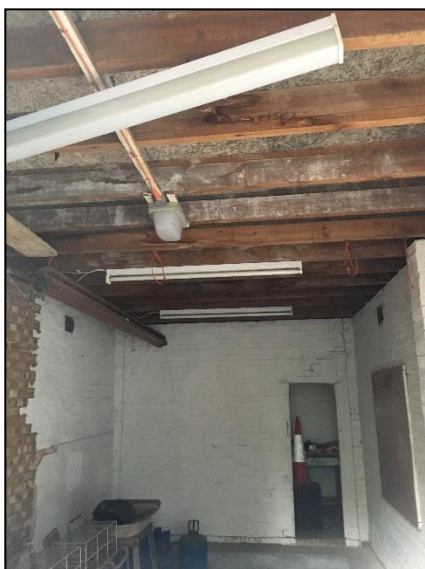
Photograph 18: Interior of building 2
