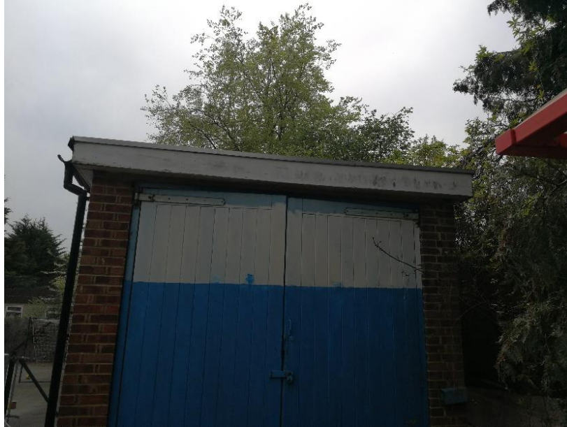
Photograph 17: Rear door to Building 2 on the Application Site.
