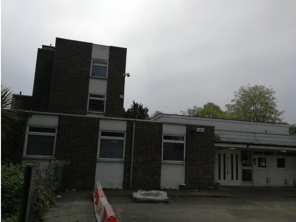
Photograph 2: View of hardstanding and northern elevation of Building 1 at the northern end of the Application Site.
