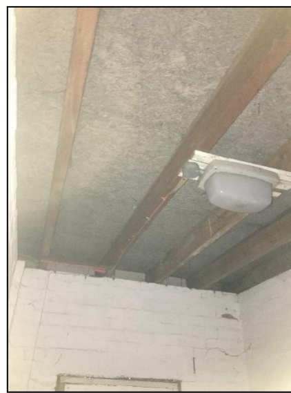
Photograph 19: Interior of building 2
