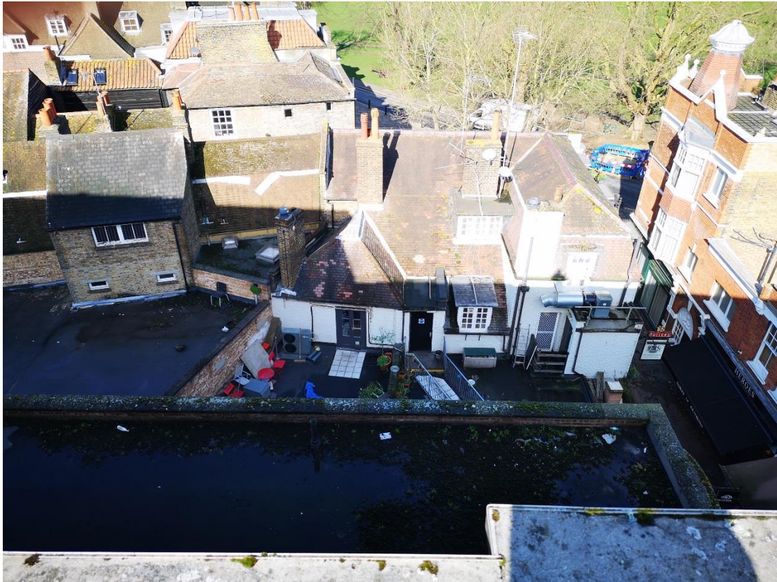
Figure 8 - View from roof looking to rear of Paved Court properties
