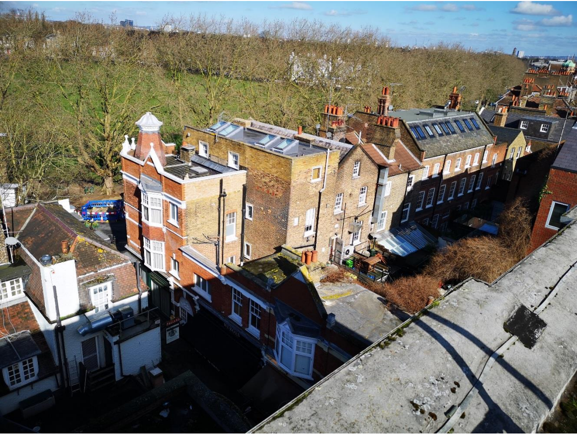
Figure 9 - View from roof towards Richmond Green
