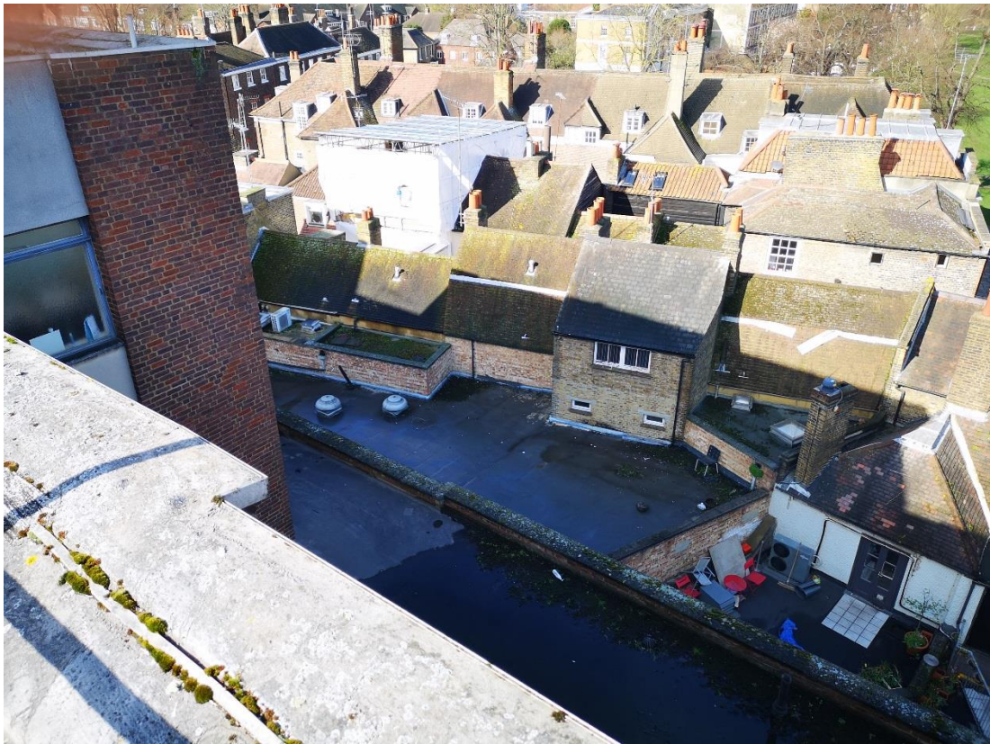
Figure 7 - View from roof looking to rear of Paved Court properties
