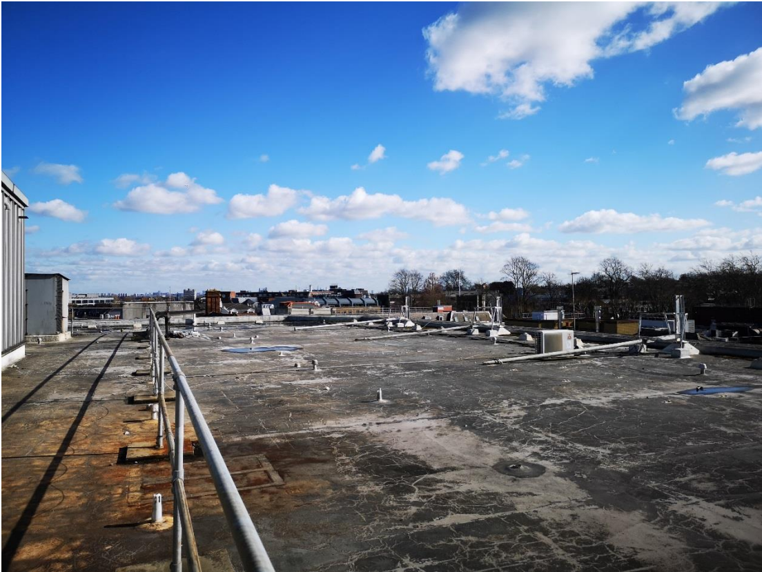
Figure 3 - View from roof
