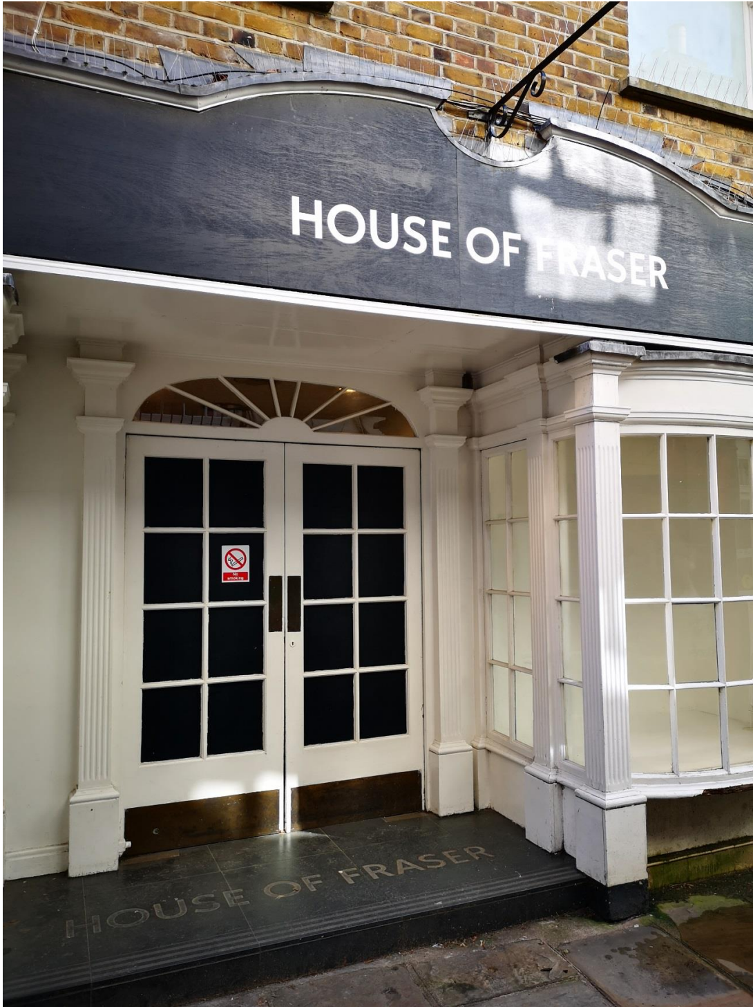
Figure 16 - Existing House of Fraser shopfront on Paved Court
