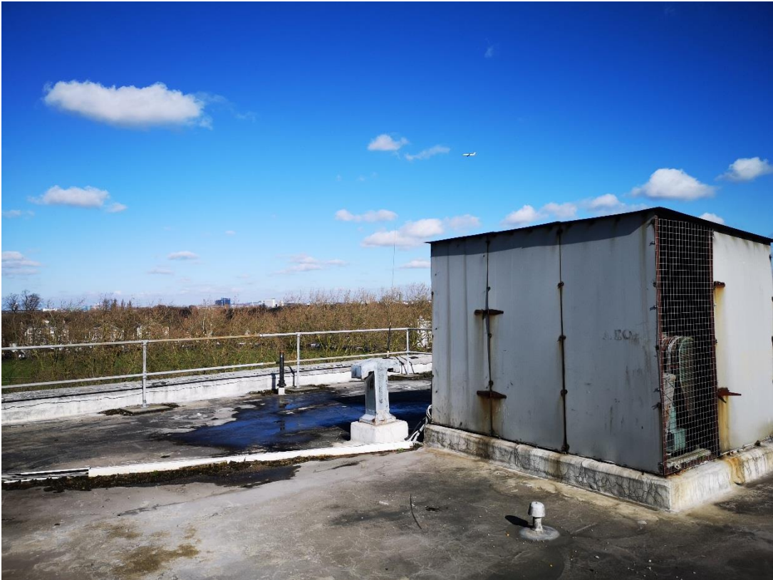
Figure 4 - View from roof / plant enclosure
