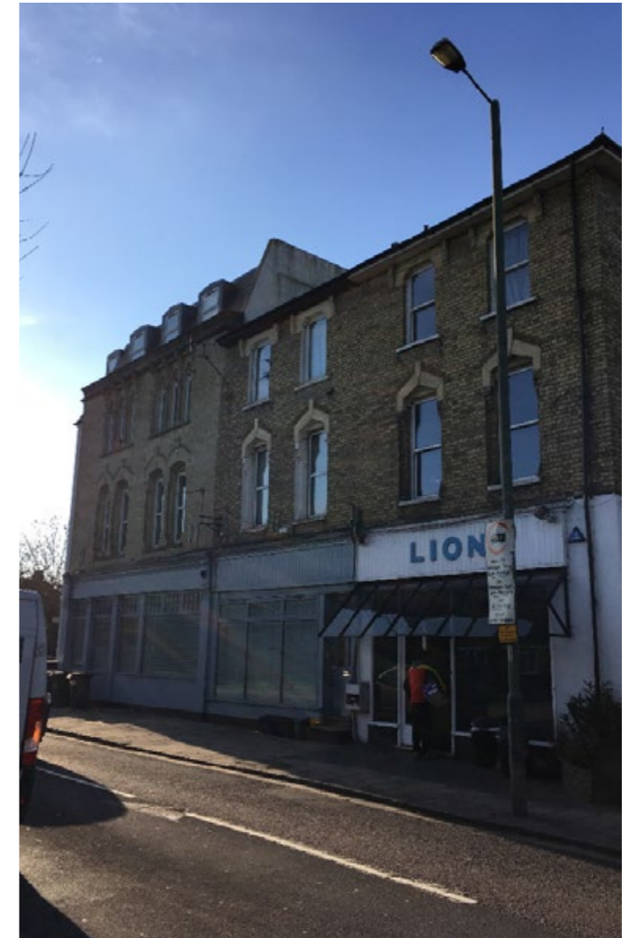
13. View of adjacent buildings on Uxbridge Road
