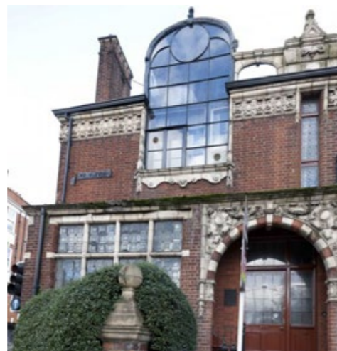
St Paul's Studios, Talgarth Road, W14
