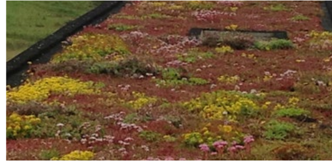
Sedum Roof Safety rails within 2m from edge
