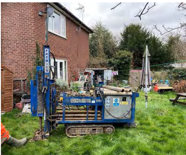
Drilling WLS3 looking east.
