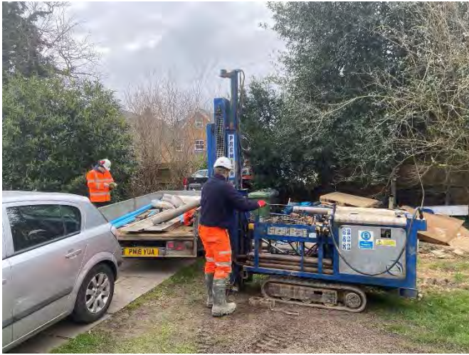
Drilling WLS1 looking east.
