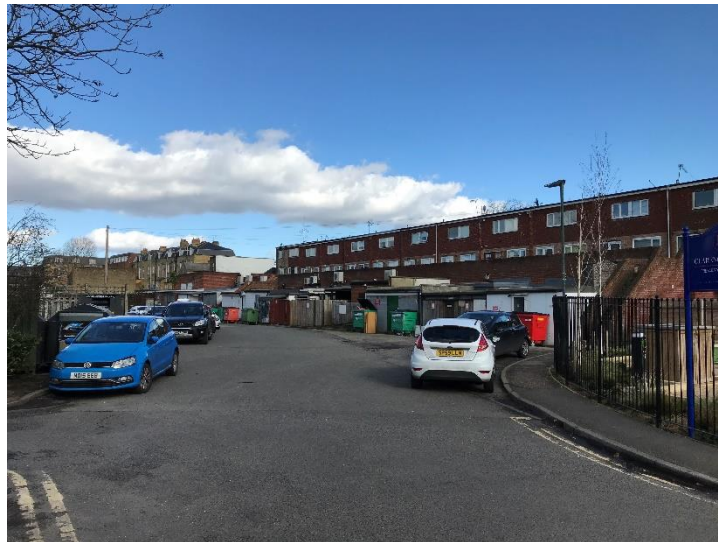
Image 1 – view towards the rear of the 1970's shops fronting High Street.
