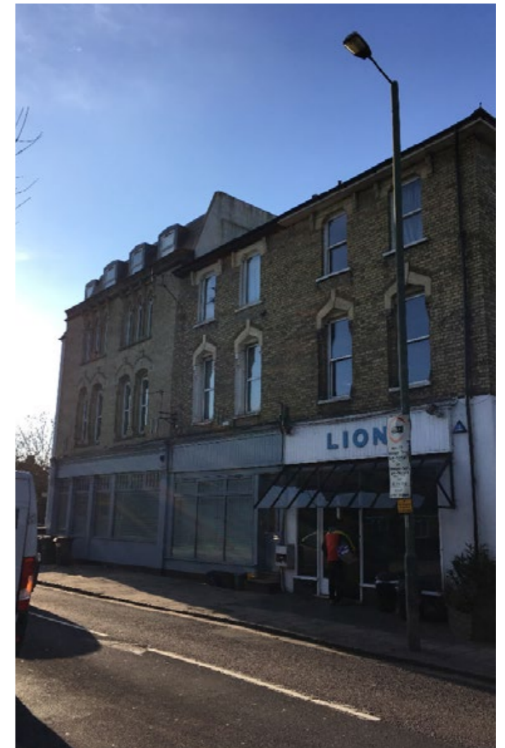
13. View of adjacent buildings on Uxbridge Road
