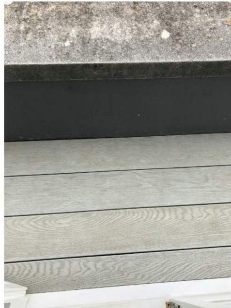
Image of decking now fitted.
