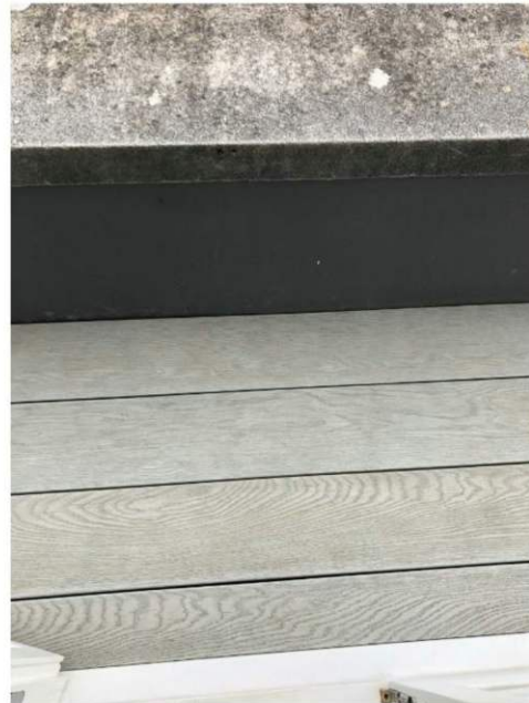
Image of decking now fitted.
