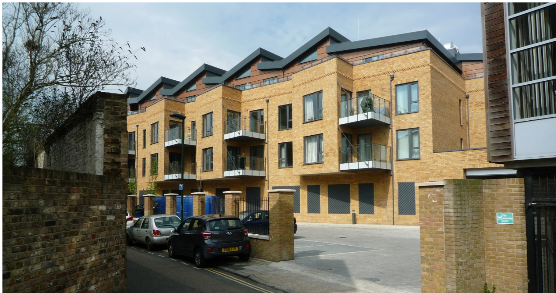
Fig. 12 - Level access approach to the building from Railshead Road.
