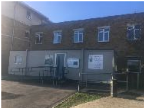
Existing temporary building and hard landscaping in front of Jii Building
