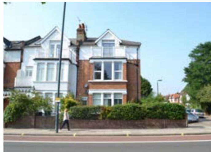
Cross Deep west side
