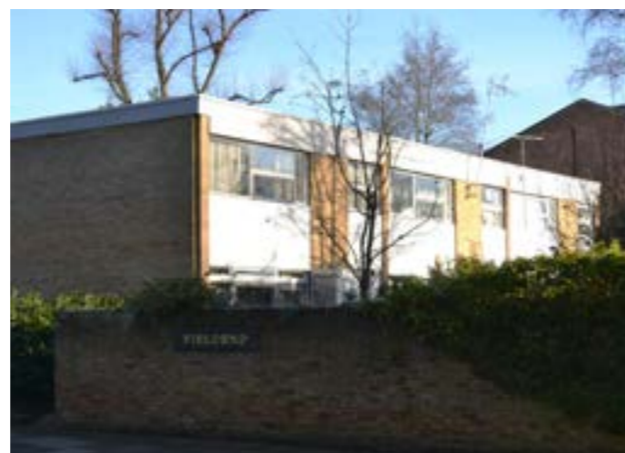
The houses are built of stock brick and have two-tone painted timber windows
