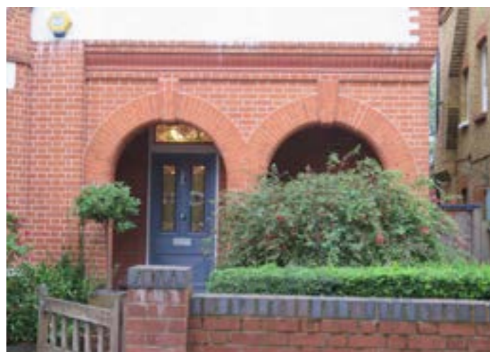
House on Waldegrave Gardens
