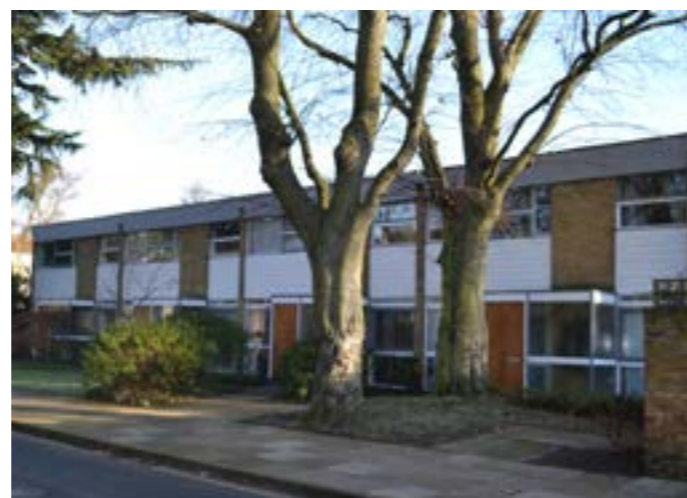
Two storey uniform terraced housing
