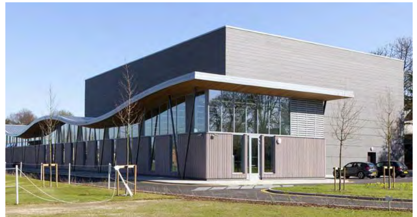
Recently completed buildings on the Strawberry Hill campus, De Marillac Halls, Dolche Vita Cafe and Sports Hall
