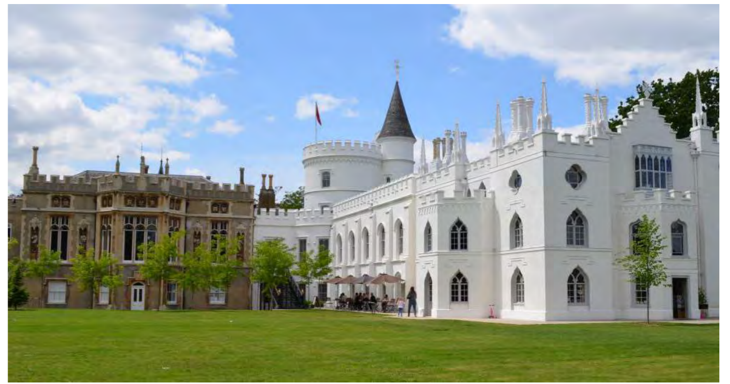
Listed buildings on the Strawberry Hill Campus, Chapel in the Woods (top) and Strawberry Hill House
