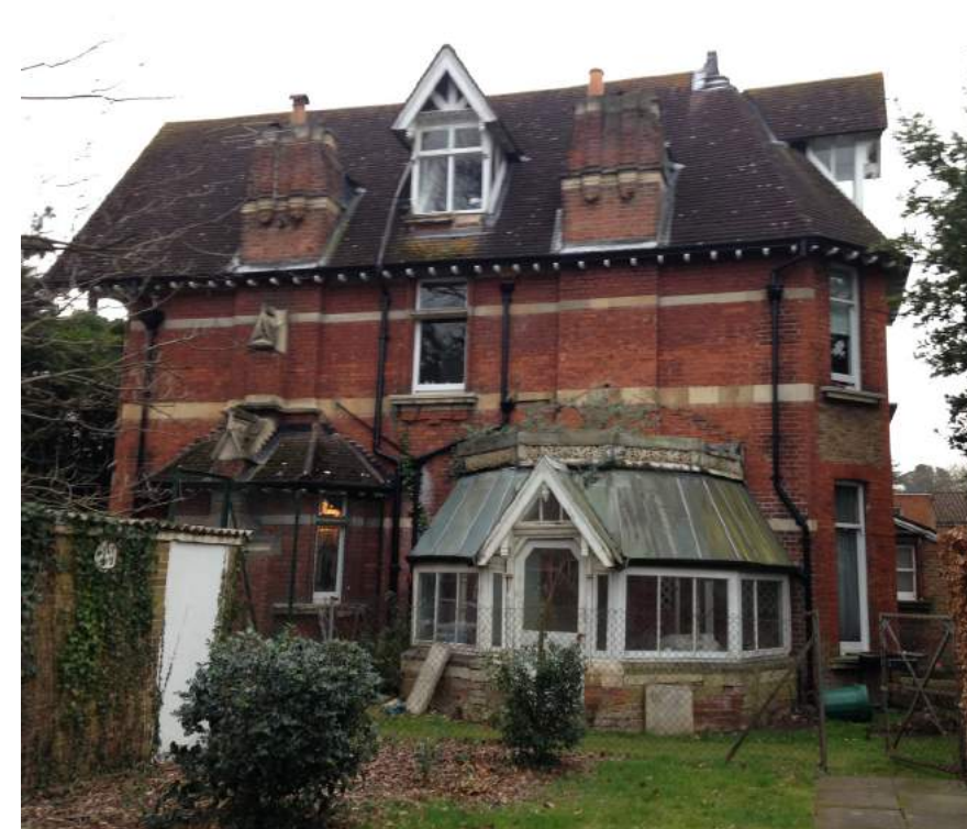
Existing buildings in poor condition
