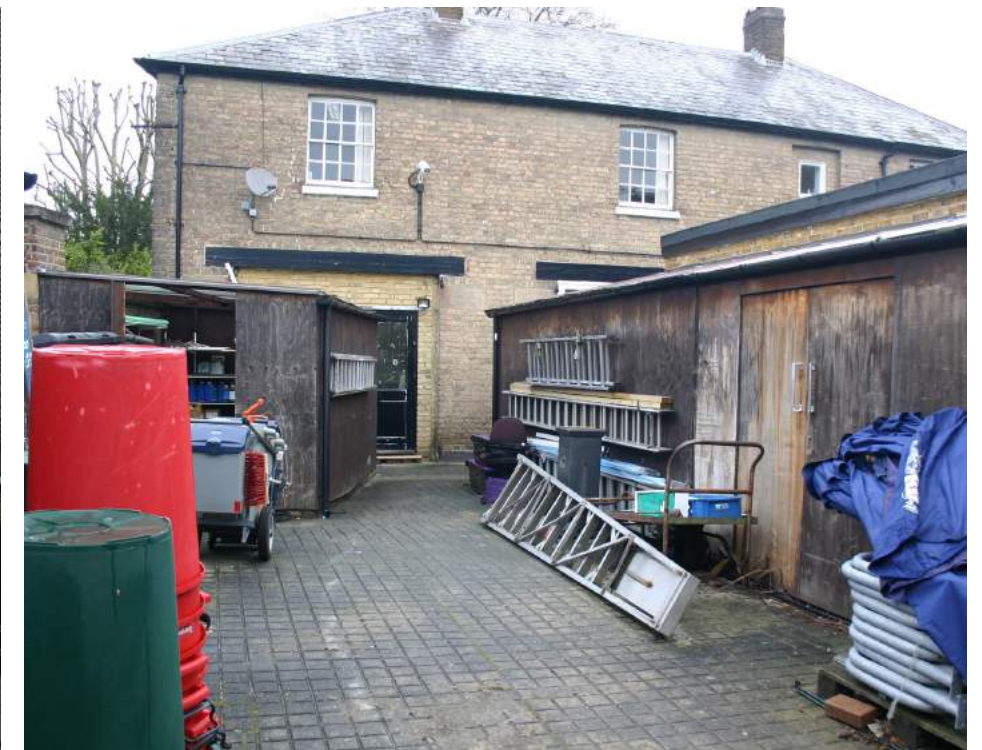
Maintenance department in E Block
