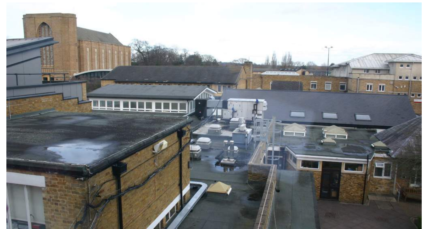
Varying roof levels across Strawberry Hill campus
