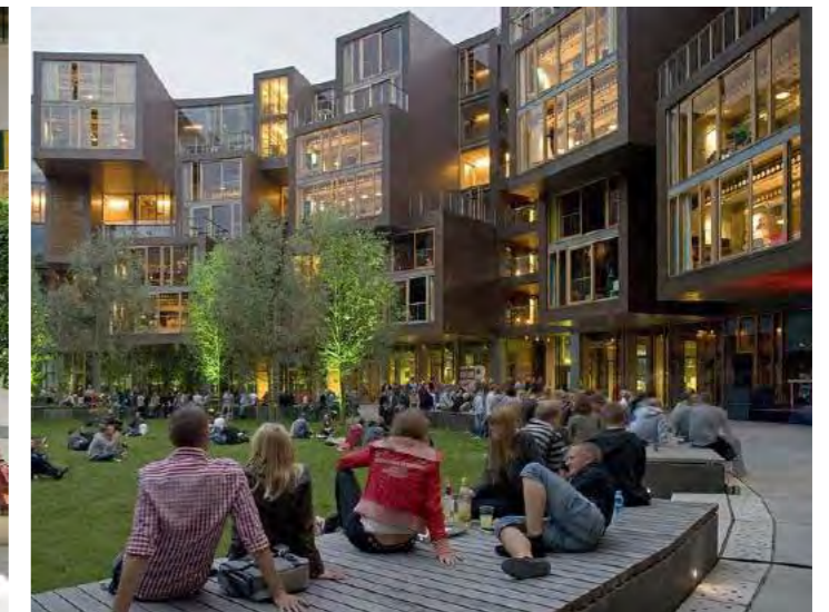
University of Copenhagen Residential Buildings
