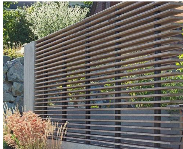
TIMBER INFILL PANELS TO EXISTING FENCE
