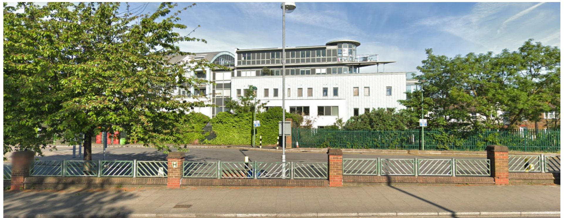
EXISTING BRICK WALL WITH PIERS AND INFILL PANELS
