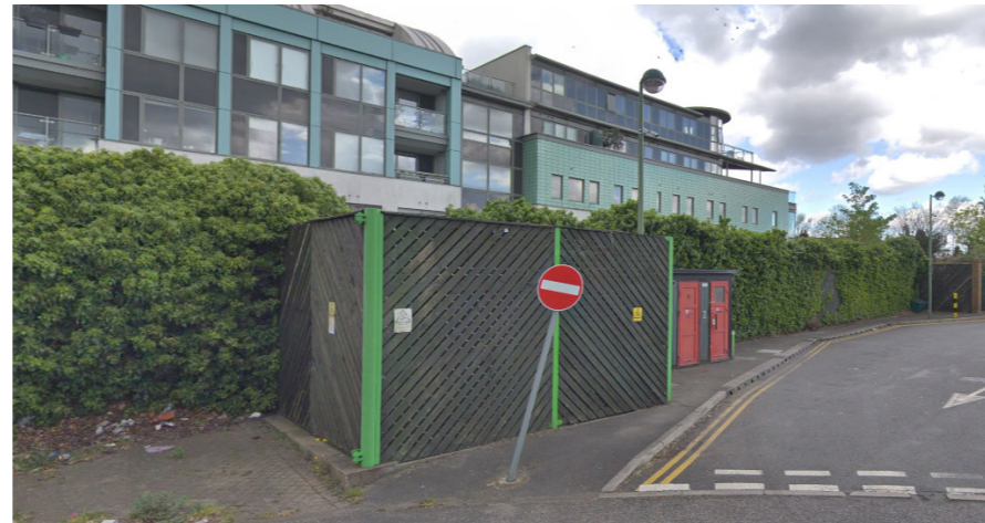
EXISTING SUB STATION ENCLOSURE
