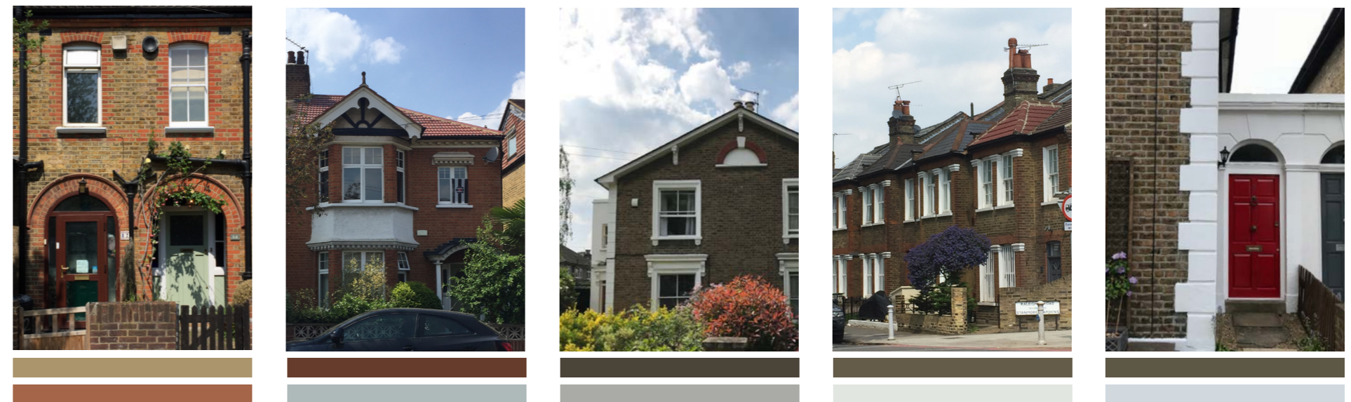
Examples of buildings within the context demonstrating the use of a contrasting colour/material to highlight the detailing on the façade
