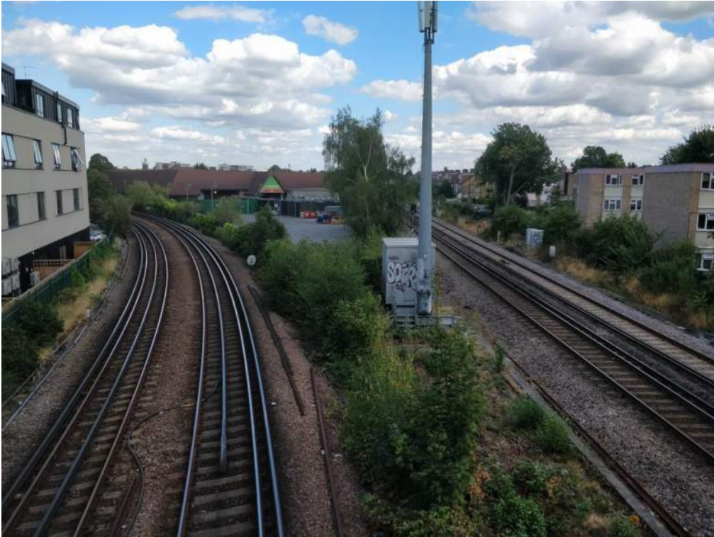
Photo 20: National Rail infrastructure
