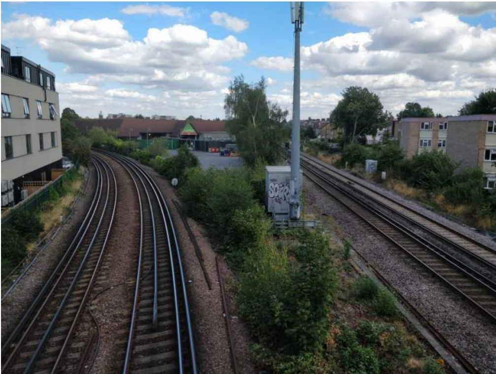
Photo 20: National Rail infrastructure
