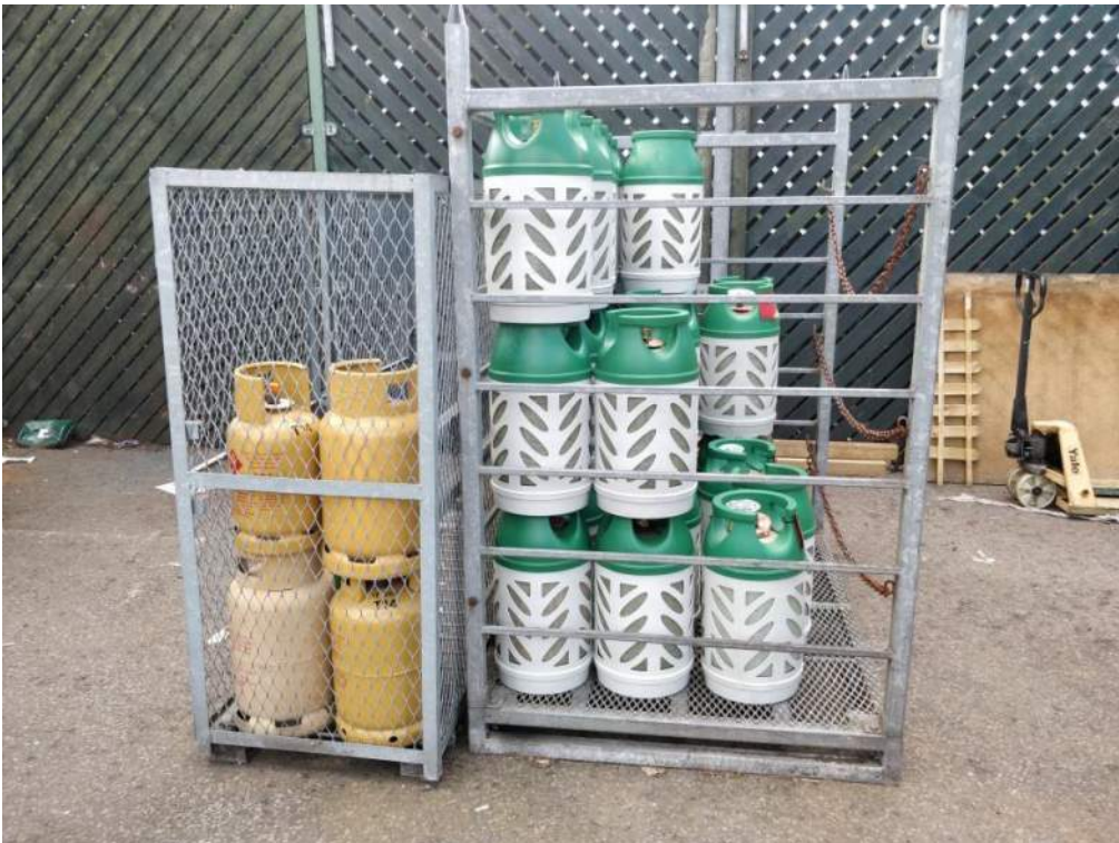
Photo 10: Gas canister storage in Homebase delivery yard
