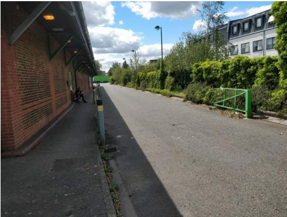
Photo 6: Access road along the western boundary of the site
