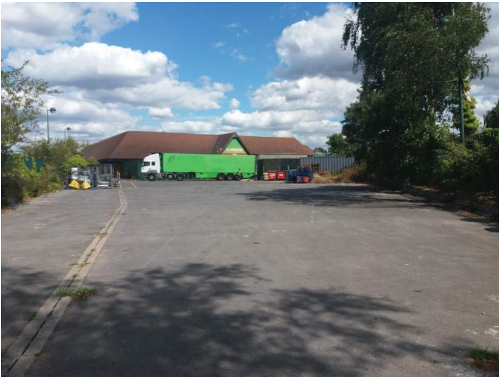
Photo 8: Delivery yard in the south-western portion of the site
