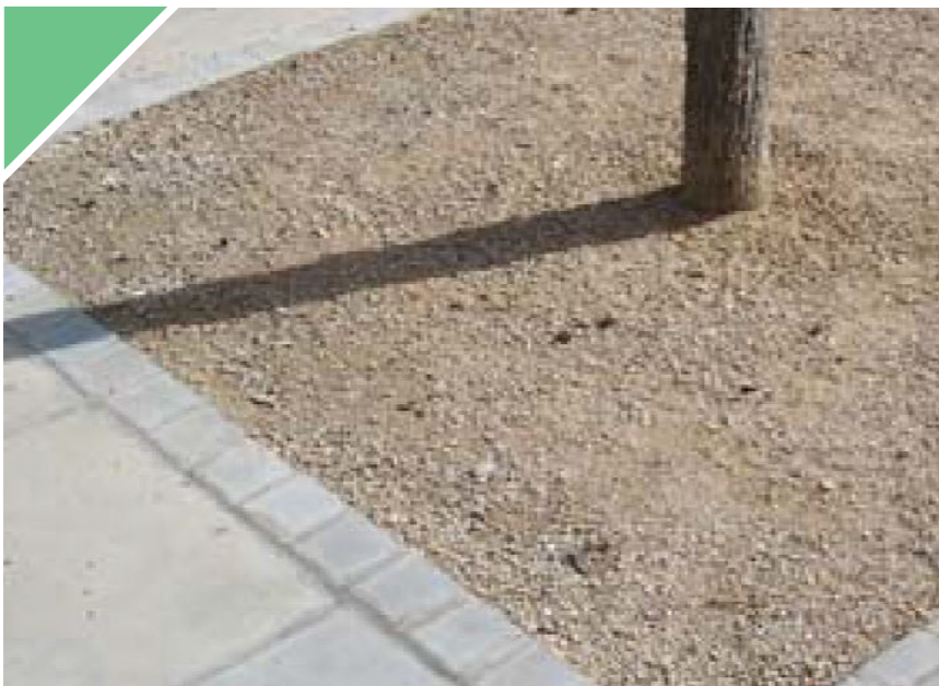
Resin bound gravel tree pit
