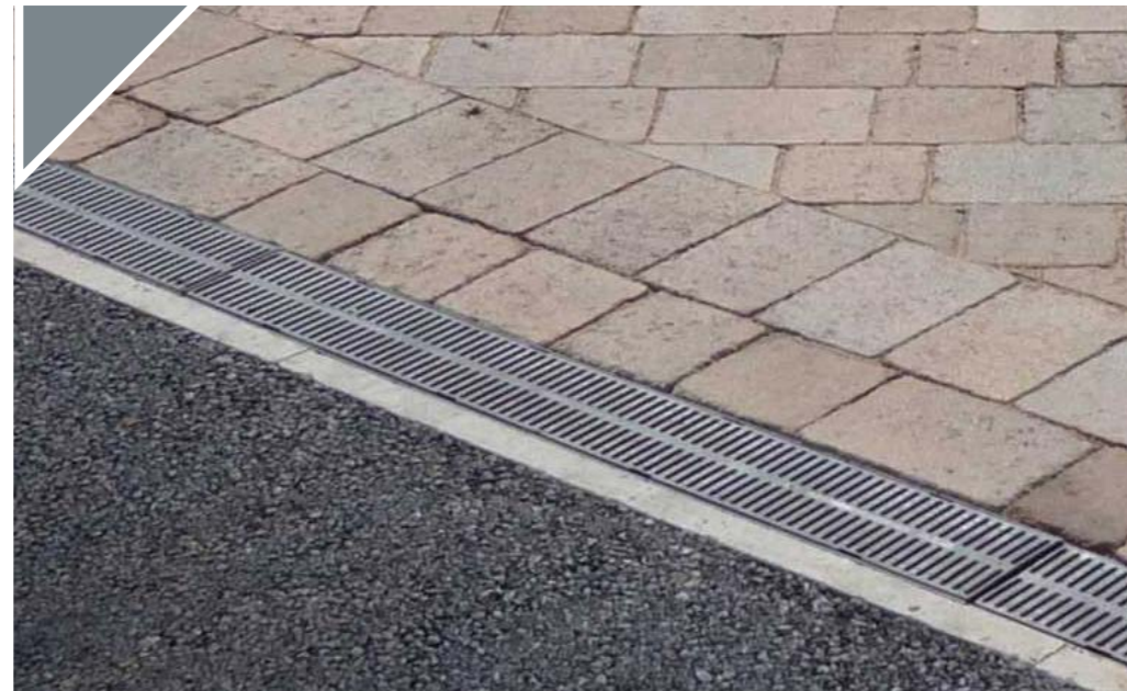
Hot Rolled Asphalt
