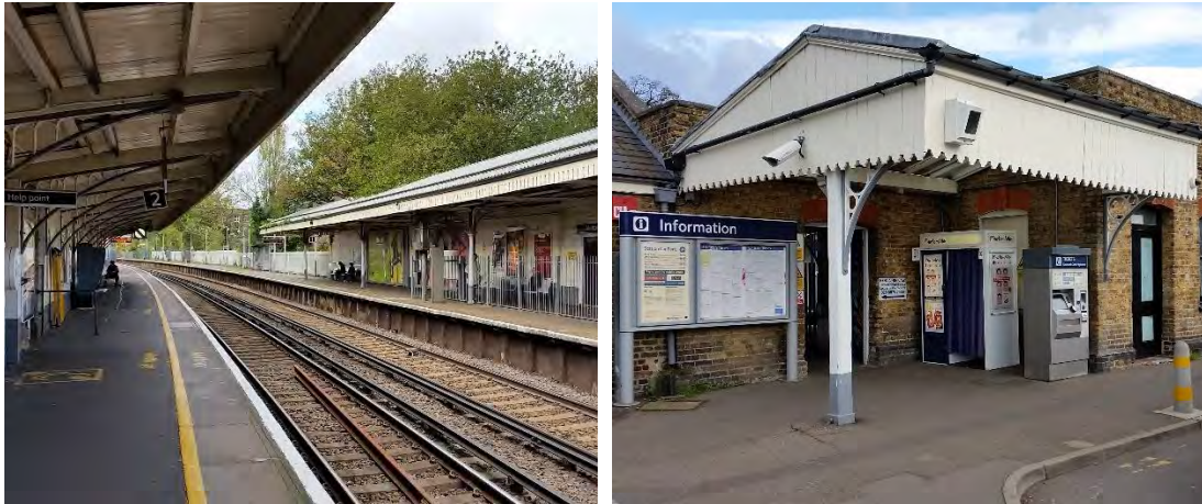
Figure 2.21 Mortlake Station Platforms and Its Southern Entrance
