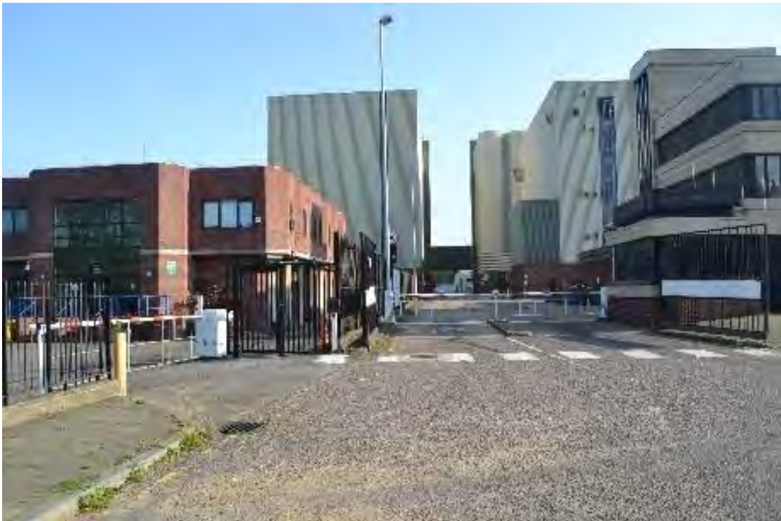
Figure 2.3: Main access to Buildings to west of Ship Lane from Lower Richmond Road; Access to Sports Ground on left
