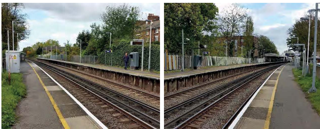
Figure 2.10: Looking West and East Along the Richmond-bound Platform
