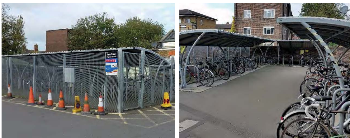
Figure 2.4: Secure, Covered Cycle Parking at the Station's Southern Entrance
