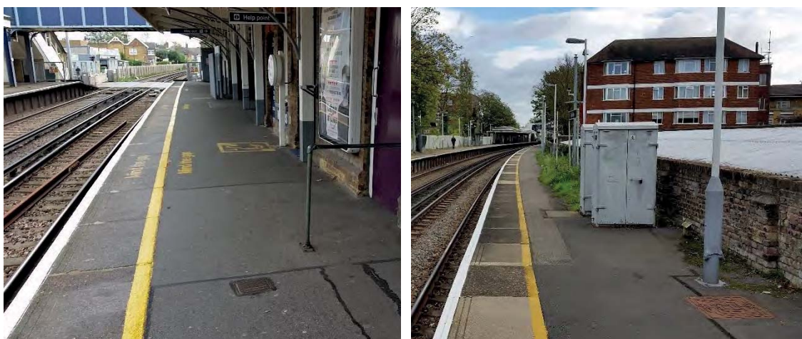
Figure 2.9: Looking East Along the Richmond-bound Platform
