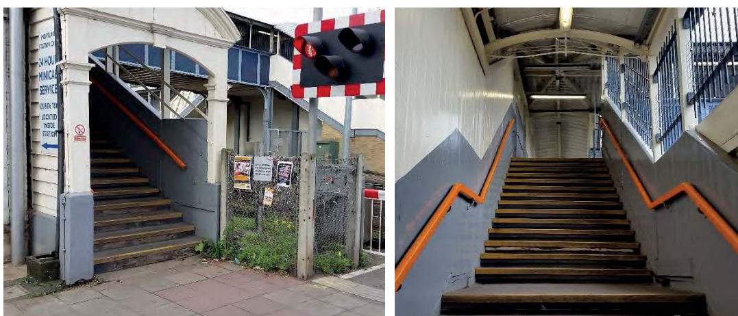
Figure 2.12: The South-Western Staircase (on Sheen Lane) Leading to the Footbridge
