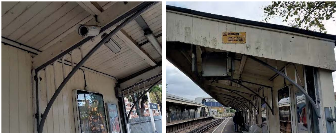
Figure 2.15: CCTV cameras on the Westbound Platform
