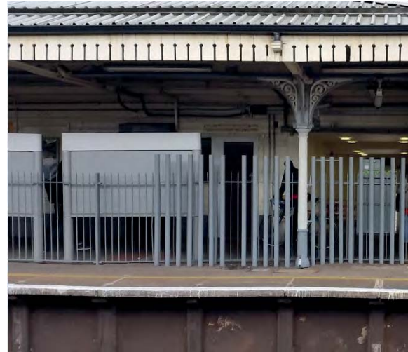
Figure 2.16: The Platform Baffles As Passengers Enter the Eastbound Platform
