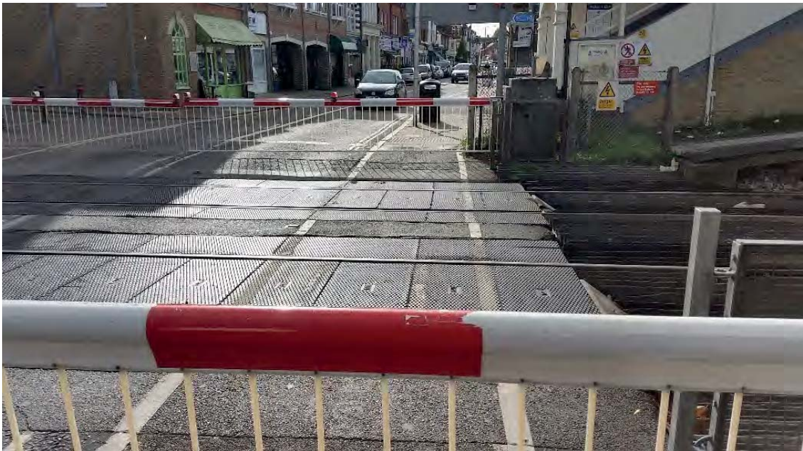
Figure 2.4: The western footpath across the level crossing
