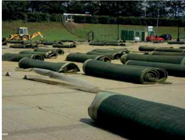
Rolled carpet ready for removal
