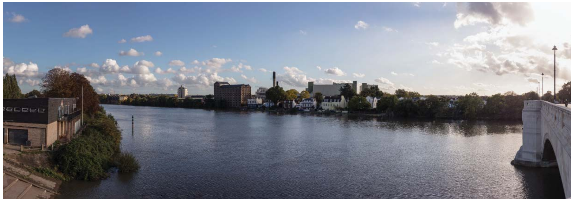
Existing view of site from Chiswick Bridge
