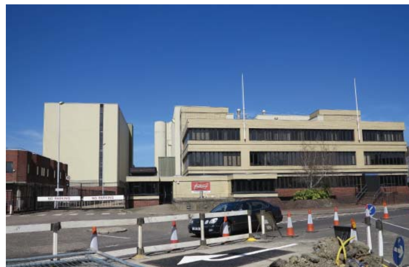
Existing office block
