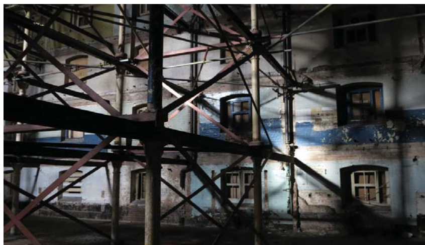
Scaffolding inside former maltings building
