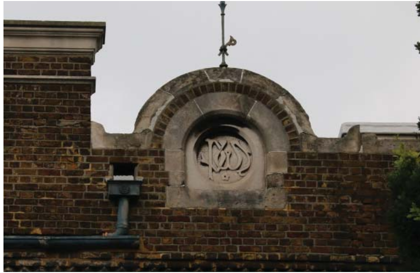
Decorative element on South elevation of existing former bottling building
