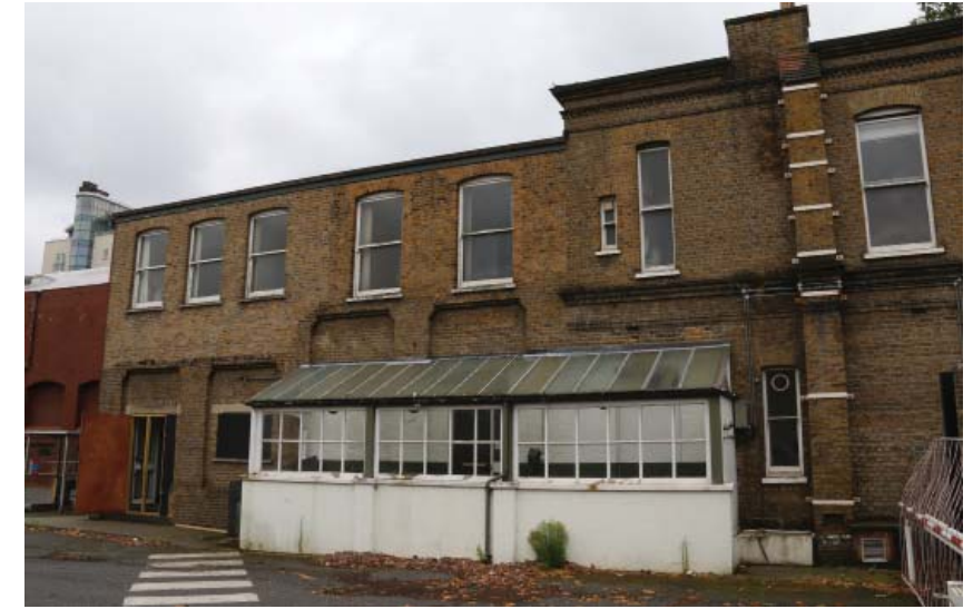
Existing North elevation of former hotel building
