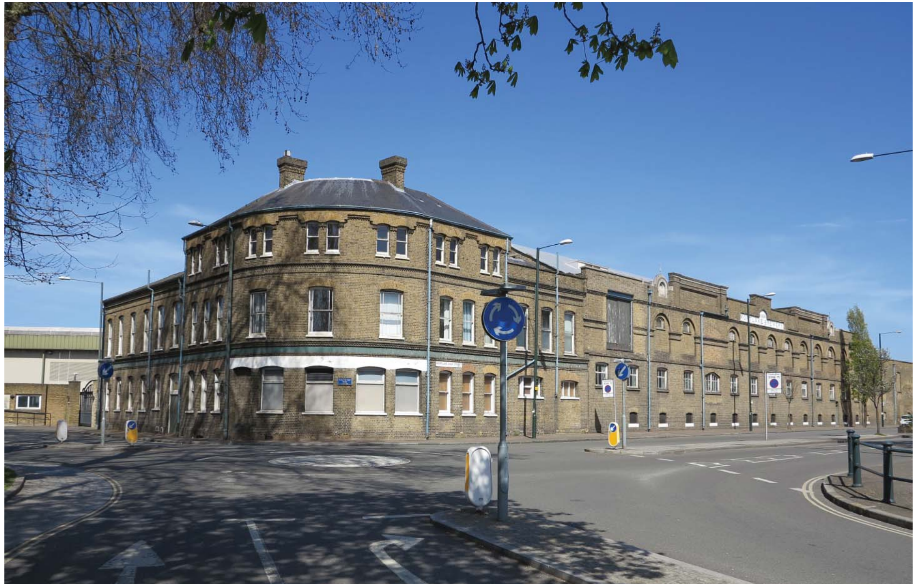
Existing former hotel and bottling building
