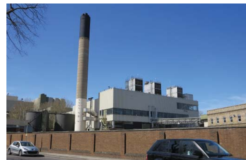
Existing power/ boiler house
