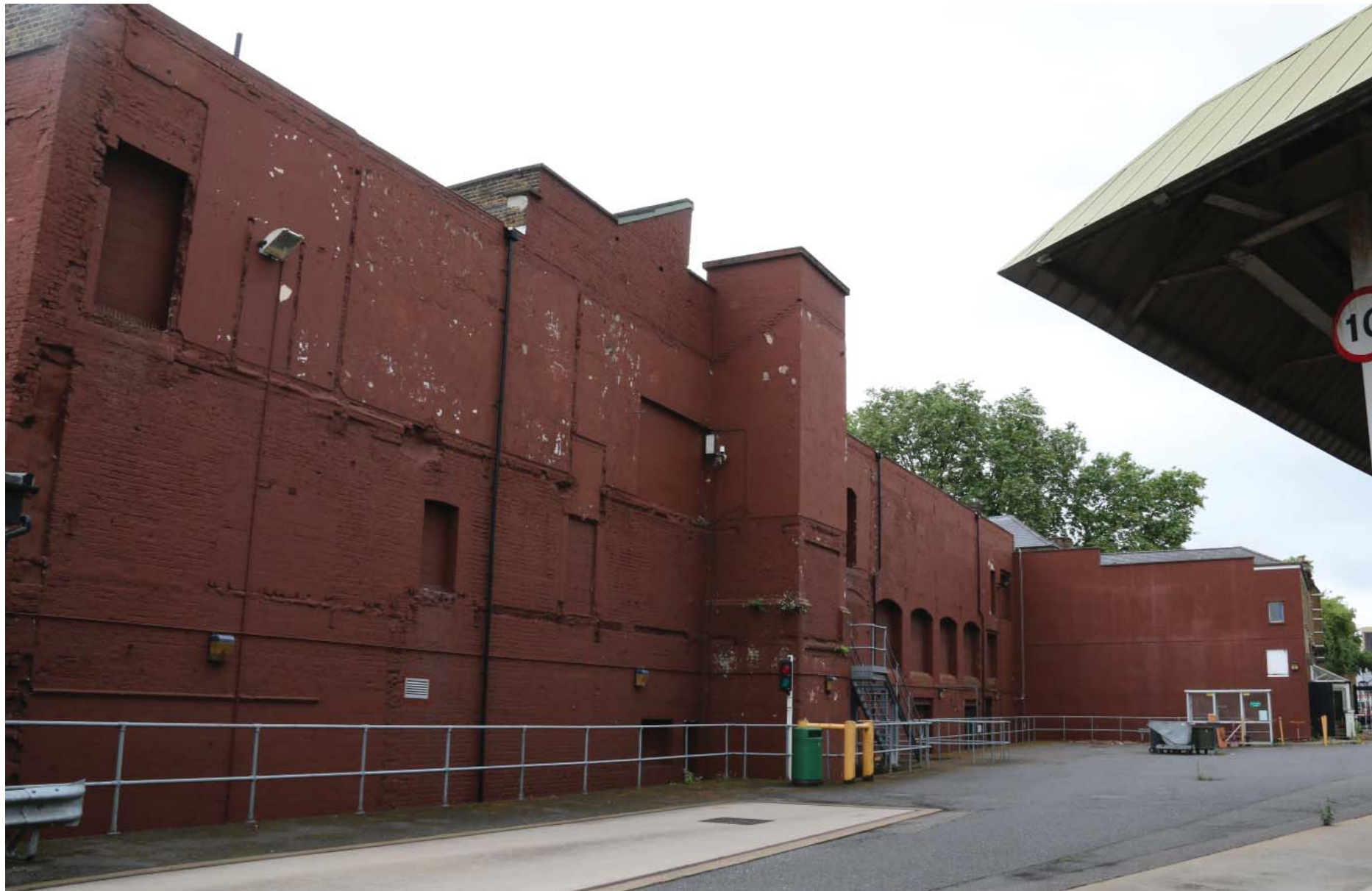
Existing North elevation of former bottling and hotel building.
