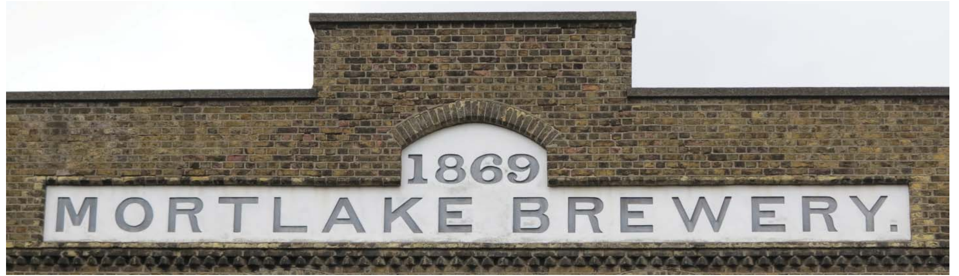
Date stone on existing South elevation of former bottling building
