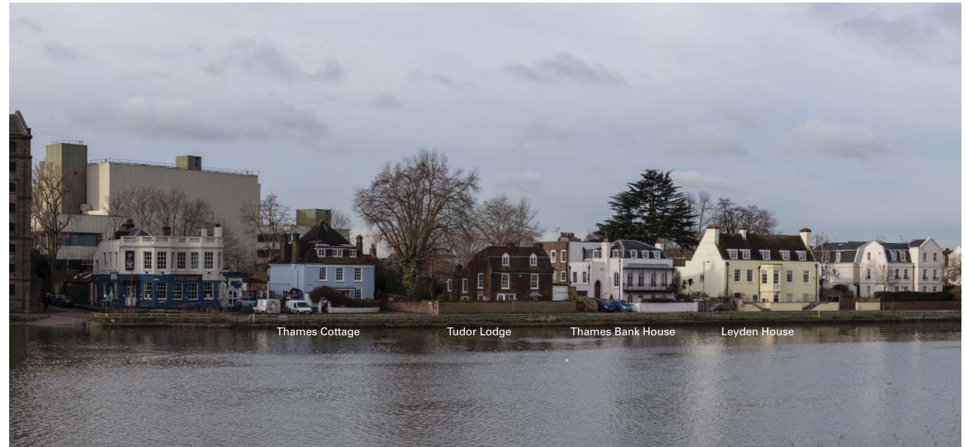
Photograph showing Thames Cottage, Tudor Lodge, Thames Bank House and Leyden House
