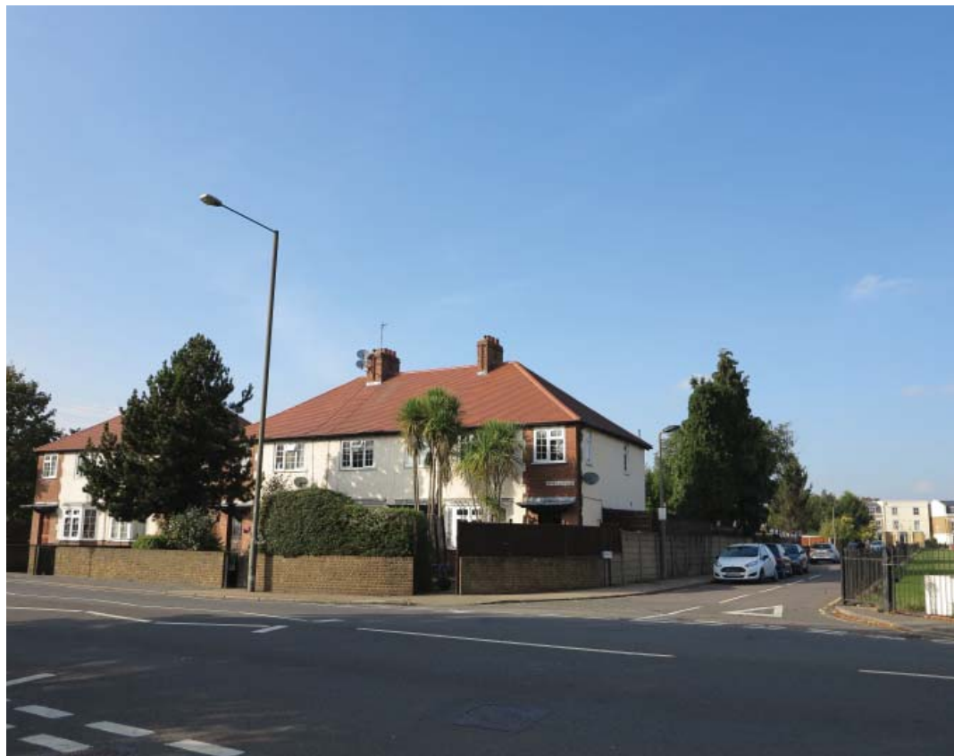
View of junction of Williams Lane with Lower Richmond Road, showing former Watneys Brewery employees housing.
