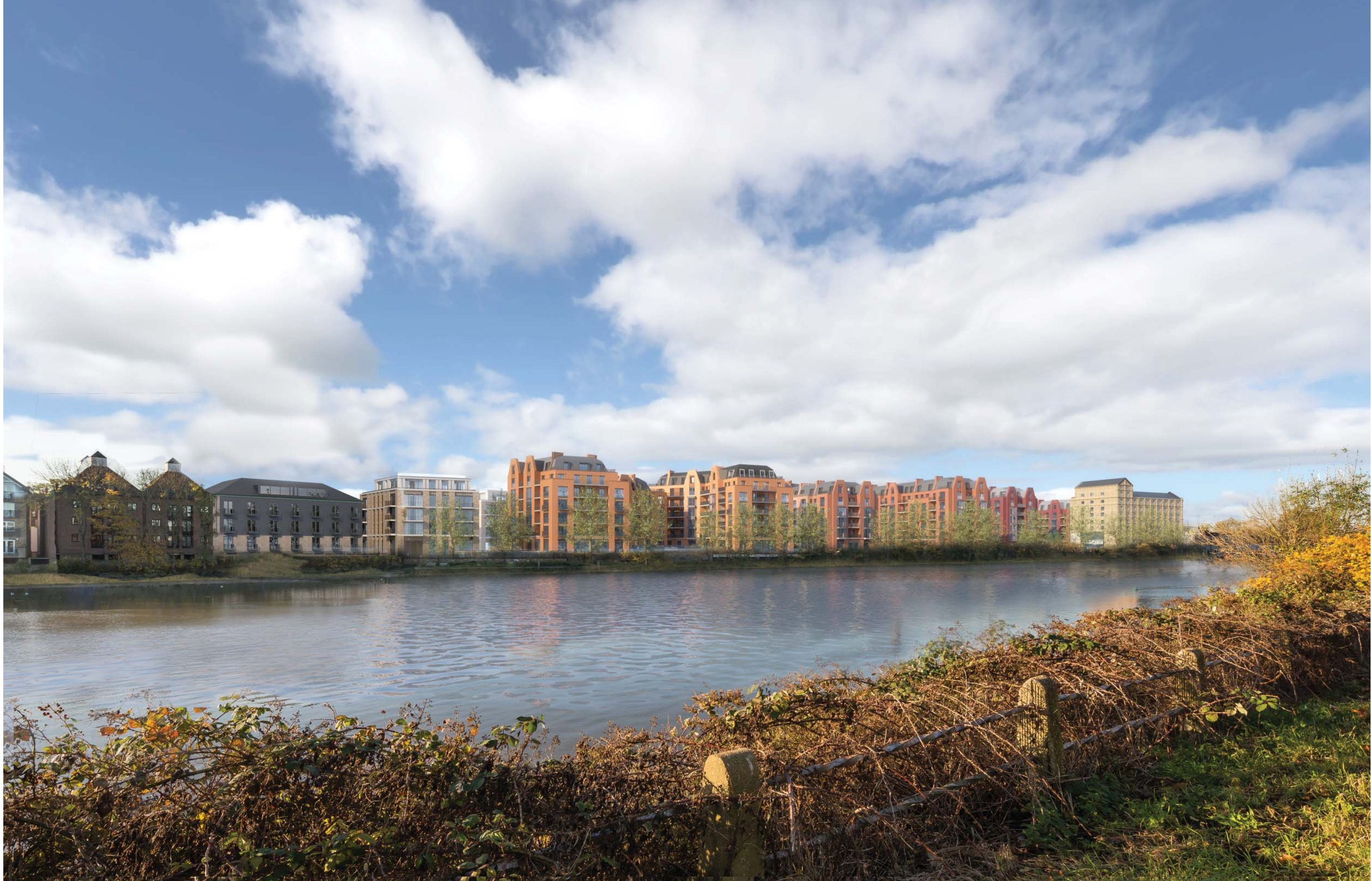
View from north east
