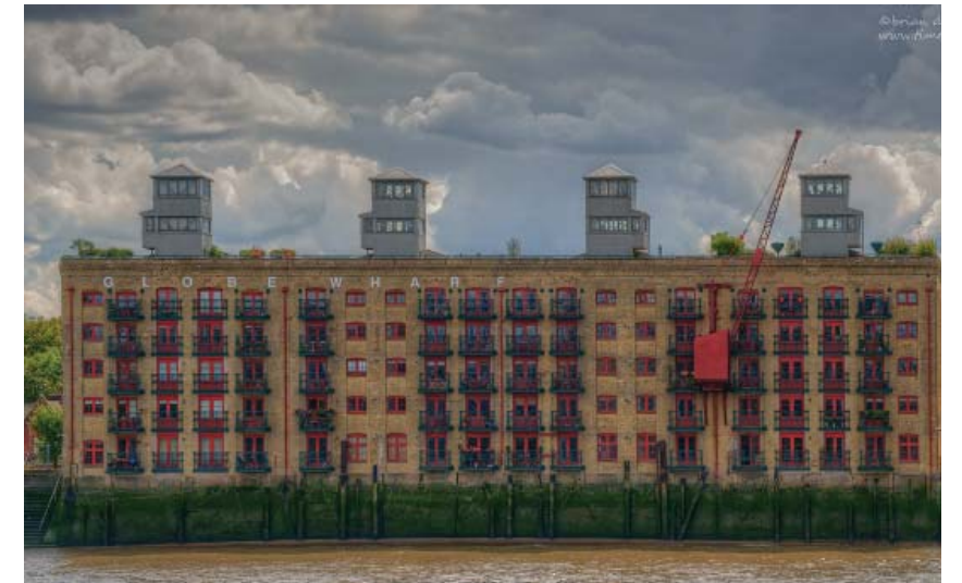
Globe Wharf - adapted former warehouse
