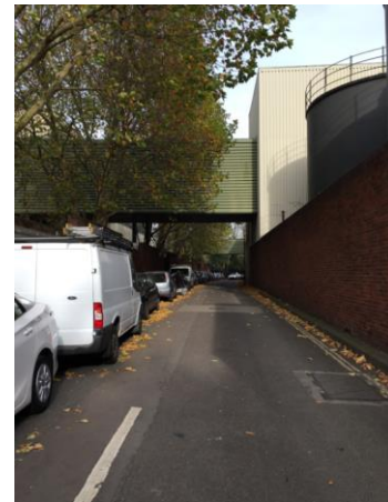
View South Along Ship Lane
